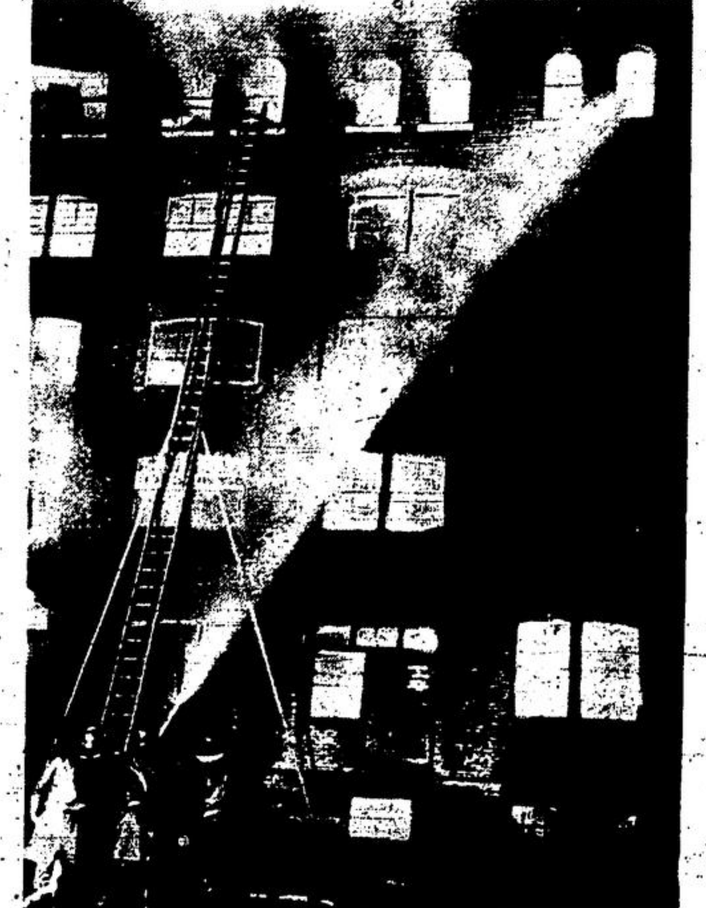
Three firemen were overcome as a result of the $75,000 fire which swept the fifth floor of the Micholias factory building in Toronto. Several other firemen received minor injuries from falling glass and debris, but remained on duty during the most grueling fight in the recent fire history of Toronto.
