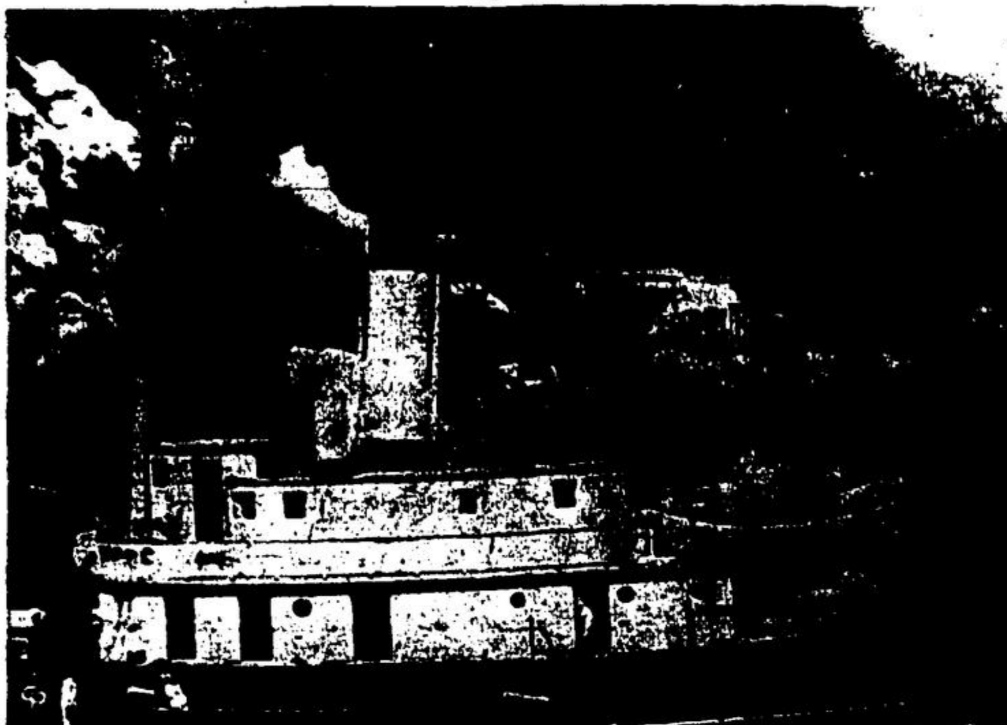
Vancouver's waterfront was turned into a raging inferno by a fire which wiped out one pier, injured five firemen and did $1,500,000 damage. All available fire-fighting equipment was pressed into service before the fire was brought under control. The fire tug Nanooce is shown here vainly attempting to stem the flames with its fireline.
