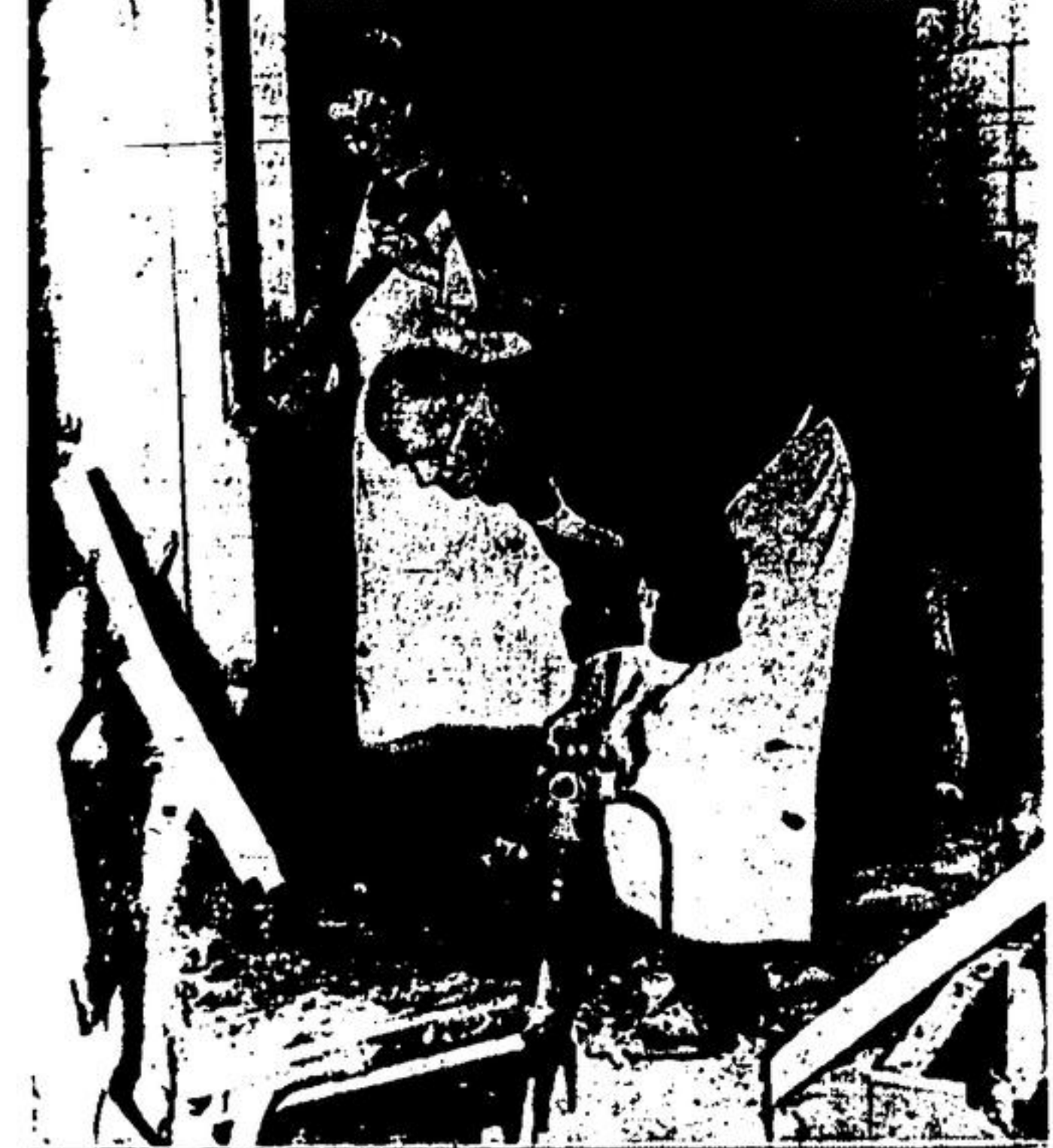
Pictured at work with a pneumatic drill is Brother Peter, first monk to start work on construction of the beautiful building that is the Benedictine Abbey of Buckfast, at South Devon, England. The monks did all the work on the abbey which is now completed, except for the installation of a heating system, the job on which Brother Peter now is engaged. He is digging a trench in the aisle of the abbey to hold the hot water pipes. Brother Paschal stands by with his pick—just in case the modern tool gives up the ghost.
