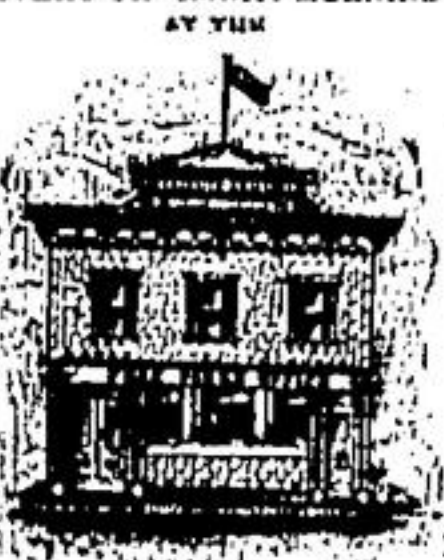
FIVE FLOOR BUILDING ACTON, ONT.
