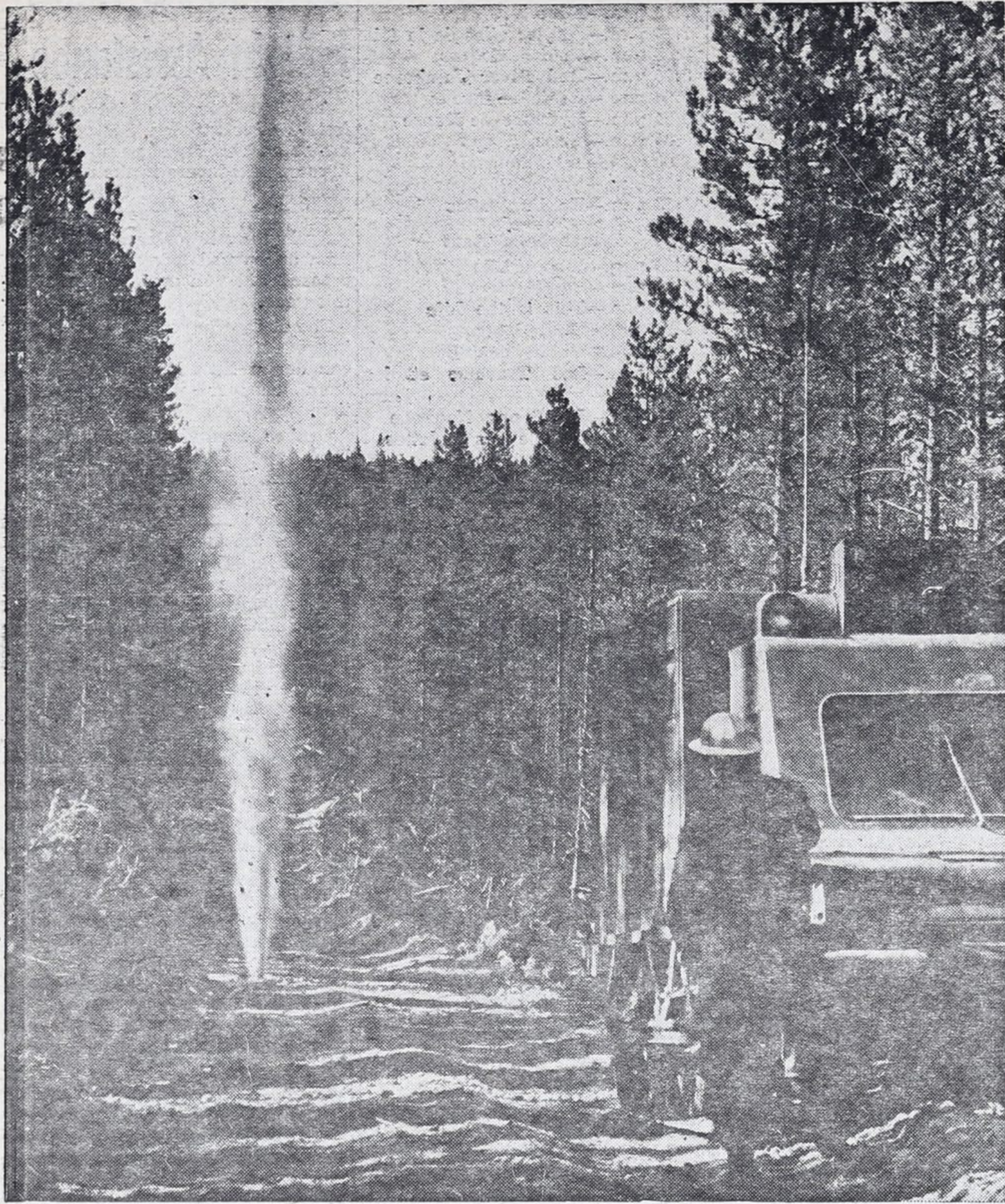
Seismic operations are presently being carried out by British American Oil on its 100,000-acre permit near Mont Joli in the Gaspé Peninsula. Here, an explosive is detonated deep in a Quebec forest and the waves are recorded on sensitive apparatus in the truck. — B-A Oil Photo
