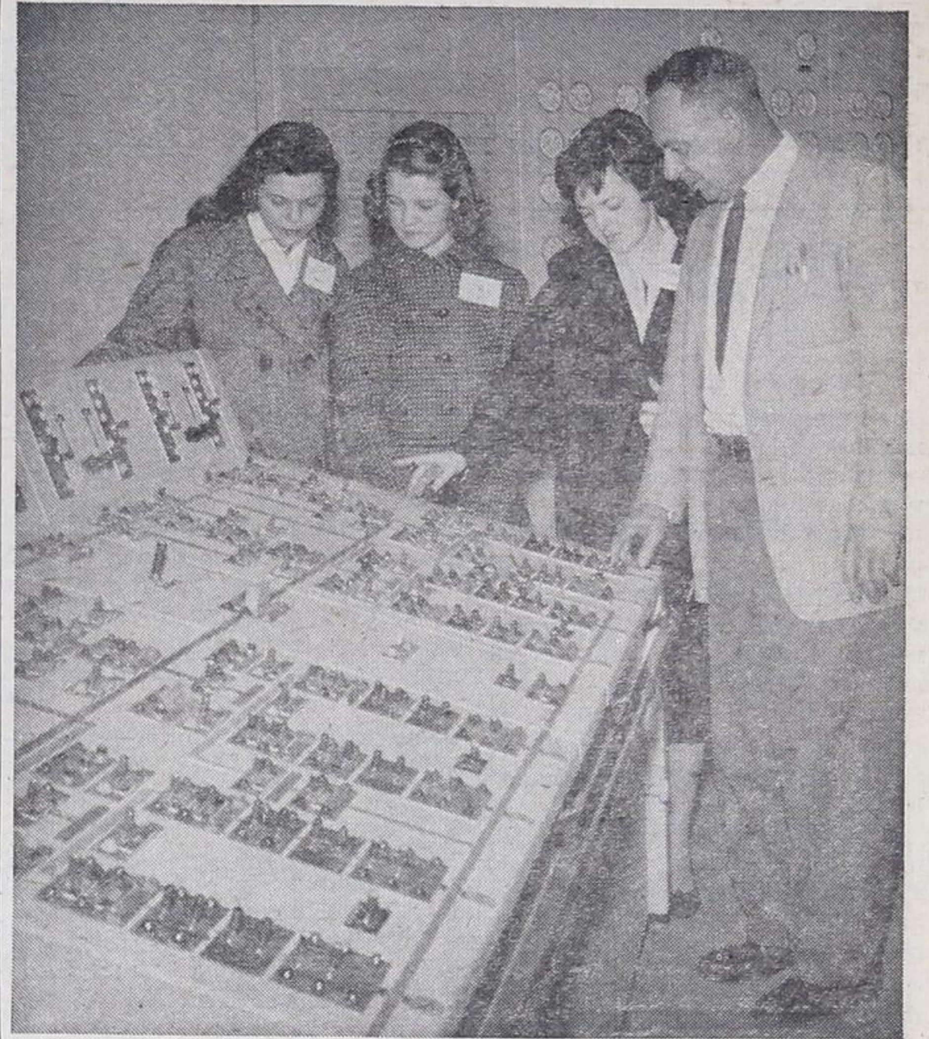
CONTROL ROOM of the Sir Adam Beck-Niagara Generating Station No. 2 holds the interest of four finalists in the secondary school section of the Ontario Public Speaking Contest. They made the day-long trip to Niagara Falls as guests of Ontario Hydro, which co-sponsored the final competition held April 5 in Toronto with the Ontario School Trustees' and Ratepayers' Association. From left: Erika Teicht, Dundalk; Carolyn Pile, Barrie, who won second prize in the prepared speech section; Harriet Conroy, Latchford; and Frank White, Ontario Hydro.
