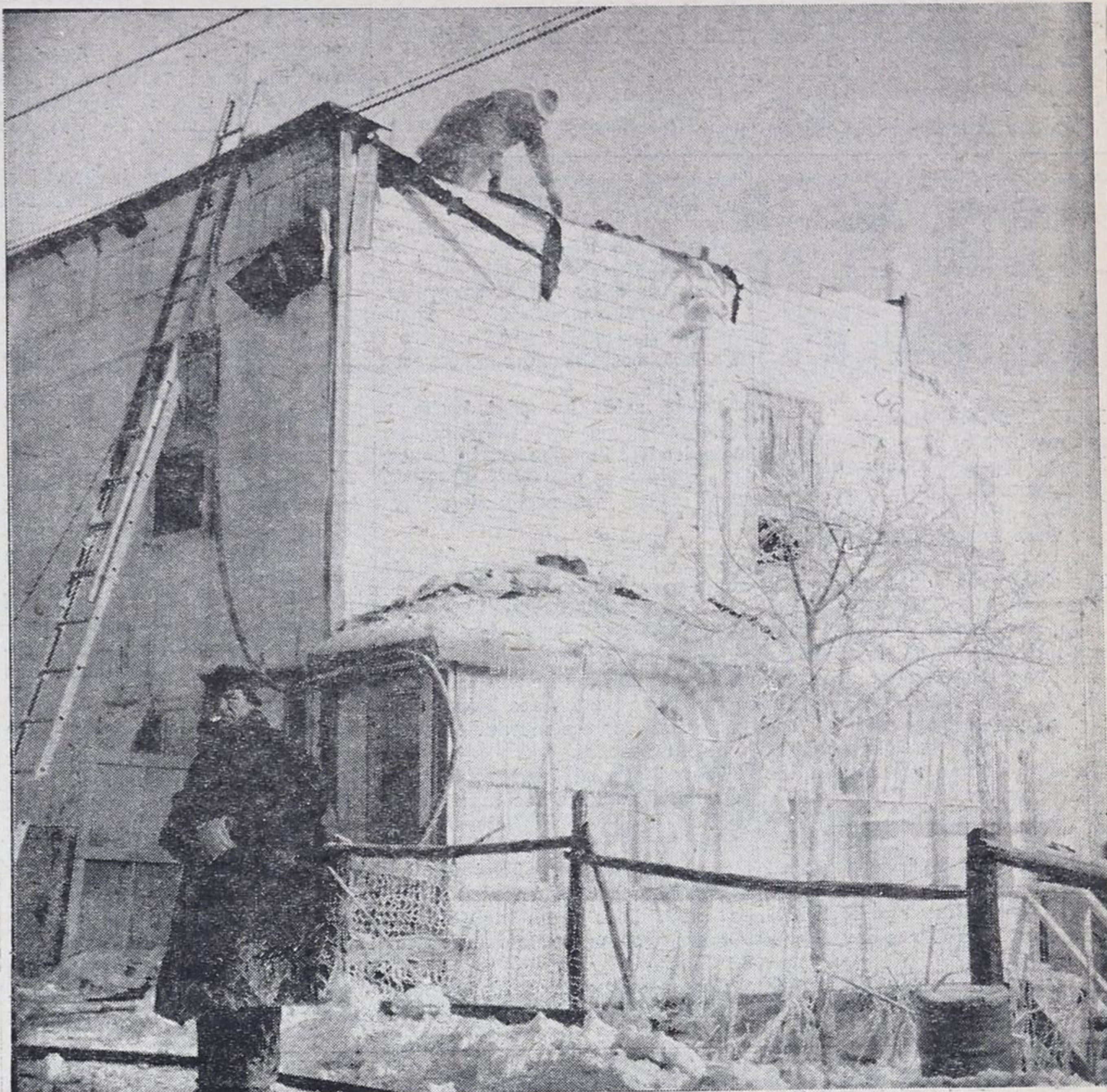
The home of Mr. and Mrs. Cezare Corbelli of Third Street, Cobalt, was seriously damaged by fire during the early hours of Wednesday morning. The fire started in the upstairs apartment occupied by Maurice Trudel, which was almost gutted. The downstairs apartment was badly damaged by smoke and water.
