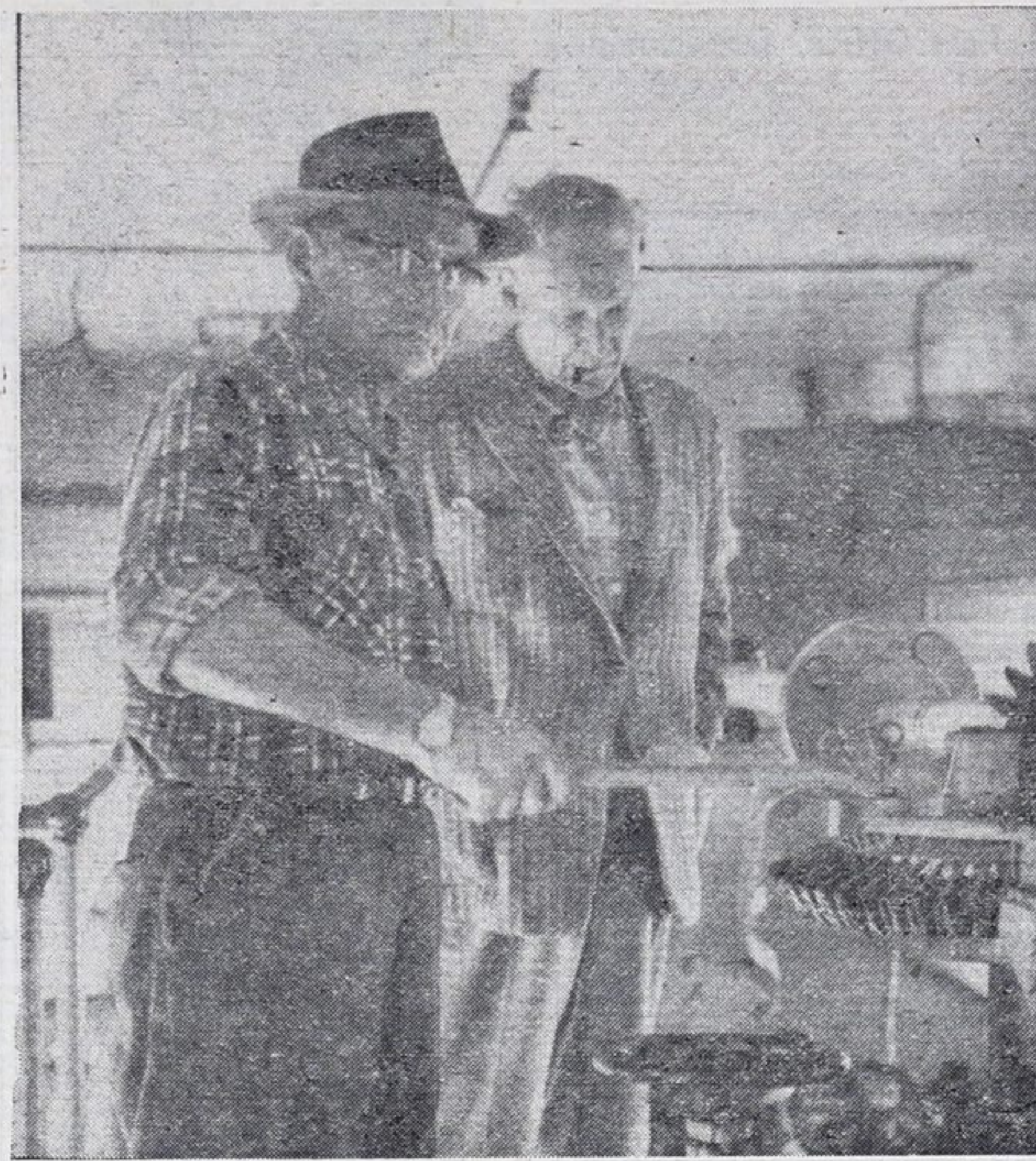
Jack Gilkes, Superintendent of the Haileybury pump house shows Water Works Chairman Chas. Camsell how the motor driven cleaners in the filters work. The filters have been one of the big expenses in this year's planned improvement program.
