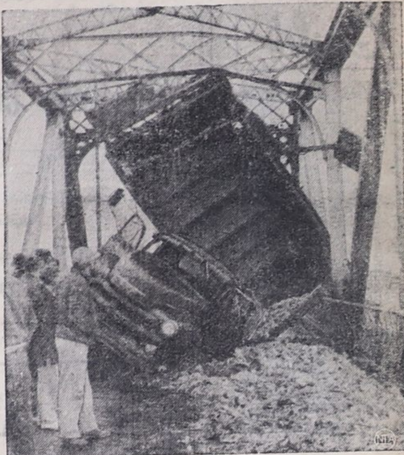
BRIDGE BLOCK —The best engineering brains probably couldn't design a more effective bridge block than this rendering company truck jammed in a bridge over Blacklick Creek. The driver, William McNamara, was not injured. How the accident to the fully loaded truck happened is open to speculation. However, there will be no speculation for the fish in the creek below as to where their next meal is coming from.
