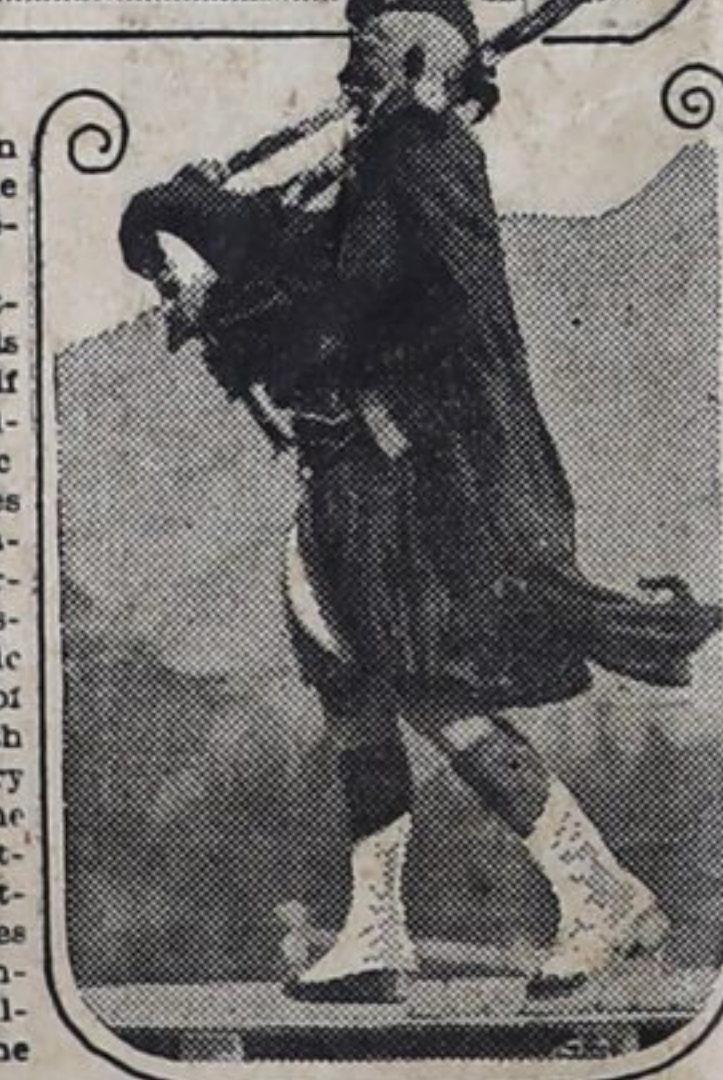
PIPING FOR FIRST PRIZE, BANFF
