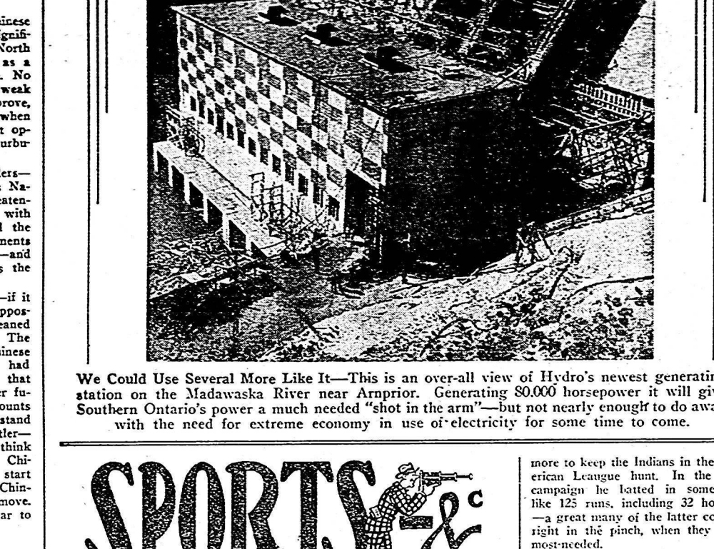
We Could Use Several More Like It—This is an overall view of Hydro's newest generating station on the Madawaska River near Arnprior.
