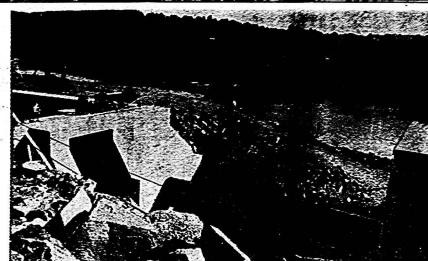
More Power-And Not Any Too Soon Either-This new hydro electric plant on the Muskoka River is different from most such installations in that it will be entirely automatic in operation, requiring only the services of a caretaker. It will add 1250 horse power to the supply for the Bracebridge area with the possibility of this amount being doubled on the completion of
