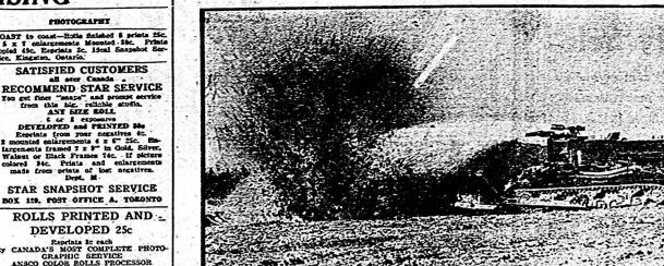
A converted Sherman tank with water nozzles instead of a cannon goes into action as a firefighting machine to defy blazing aircraft or exploding ammunition. Known as an "ammunition dump fire fighter," the remodeled land dreadnought is expected to revolutionize methods of controlling dangerous fires by permitting fire fighters to track right into the middle of the blaze with water foam, ignoring danger of falling walls.
