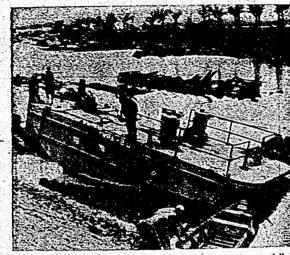
First one to be launched on the Rhine River, the "sea mule" in the photo above was backed into the water off a trailer on which it was transported 'cross-country. The "mule" was used by Allies to tow tugs and haul heavy engineering supplies.
