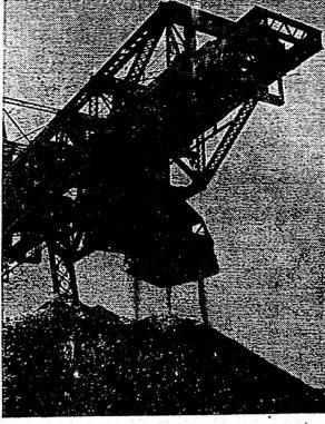
THIS huge overhead travelling bridge, equipped with 10-ton clamshell bucket, is one of two such units operating at the Canadian Pacific Railway Company's big coal dock in Fort William, Ont, where 1,224,000 tons of American bituminous coal were handled during the Great Lakes navigation season in order to relieve western Canada's threatened fuel shortage.
