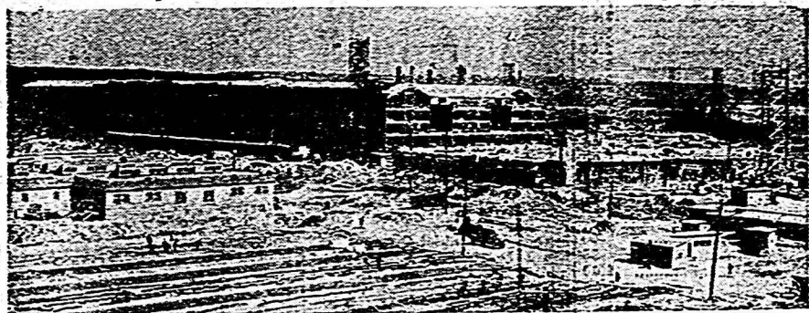
Four buildings within a building form War Department's new headquarters, under construction at Arlington, Va. Pentagonal in shape, structure will be largest office building in world.
