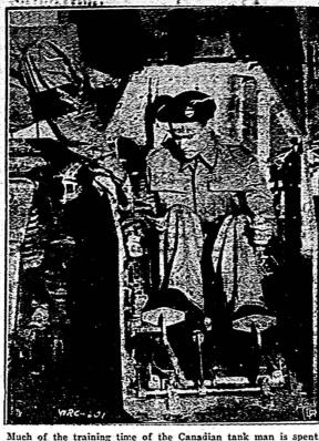
Much of the training time of the Canadian tank man is spent in the class room, where he learns all the tricks of the intricate machines with which modern war is fought at high speed. A driver is shown here as he sits in one of the special instruction tanks. These have sections cut away to reveal the action of the controls and other equipment.
