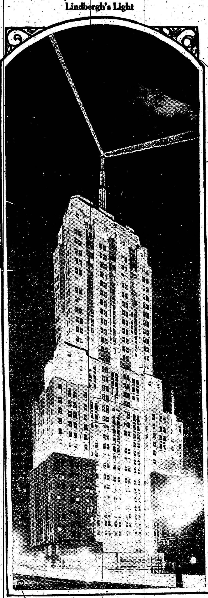
Lindbergh Beacon, most powerful searchlight in world, recently placed upon top of Palmolive building in Chicago, from where its light shaft carries for many miles.
