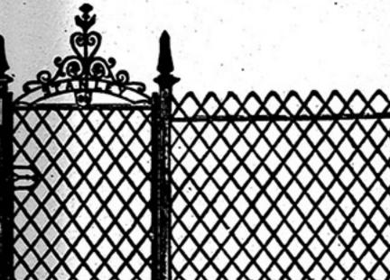
Made from 3.16 Steel Rods, with Heavy Iron Frame and Iron Foundations.
