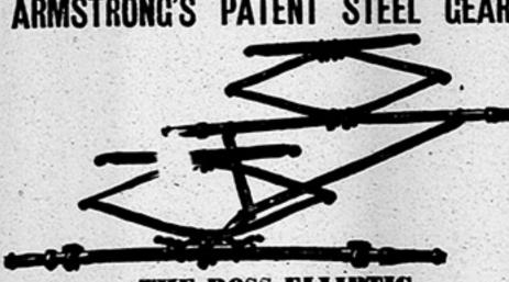
THE BOSS ELLIPTIC. All Furnished with our patent improved PERFECT SINGLE PLATE SPRINGS, three inches less open than formerly made, thus hanging the body that muchlower The taper of plates has also been entirely changed and we claim to have a PERFECT RIDING SPRING with light or full load, and one that WILL NOT BREAK. Every carriage maker should handle these gears. PRICES RIGHT Full particulars on application. J. B ARMSTRONG M'FG. CO, (Ld), Guelph, Canada.
