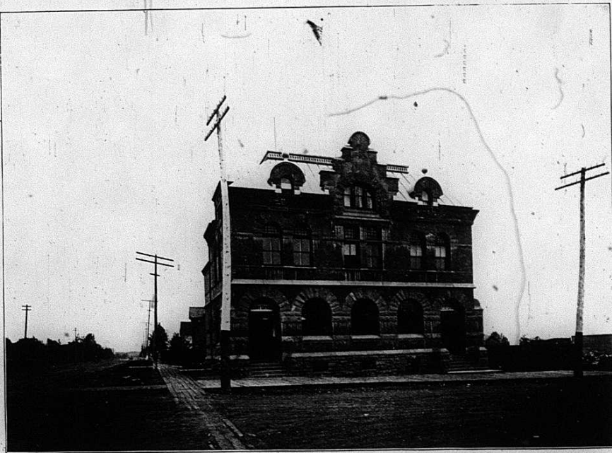
POST OFFICE, PORT ARTHUR.
