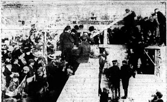
Miss Mary McKellar is shown above laying the corner stone of the John McKellar Memorial Hospital on South John Street, October 7, 1902. The $16,000 hospital was completed in June, 1903, and had accommodation for 35 patients.
