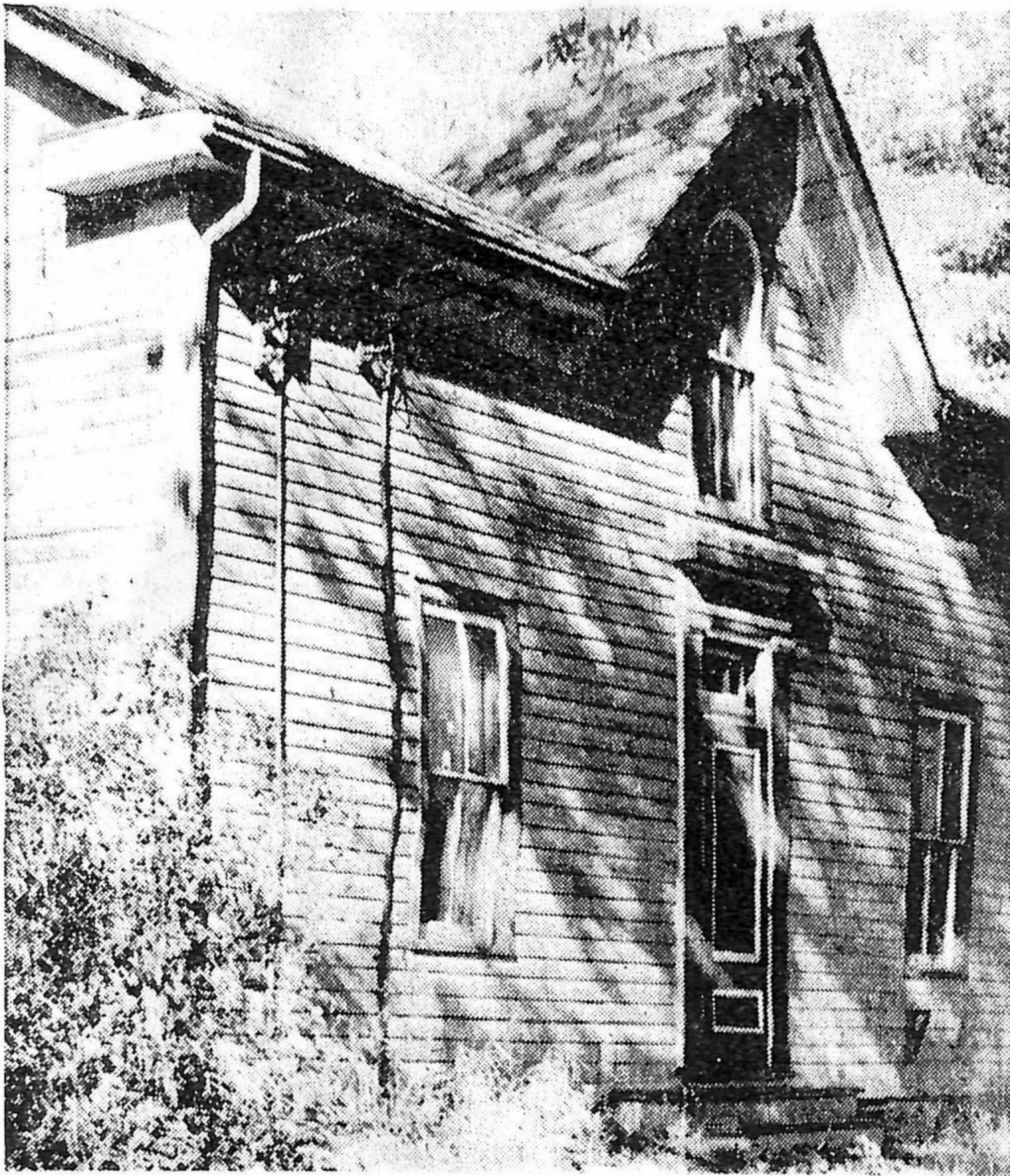
A historic marker will be erected at the home in South Dumfries Township where Adelaide Hoodless was born. She was the founder of the Women's Institute. (Photo by Marshall).
