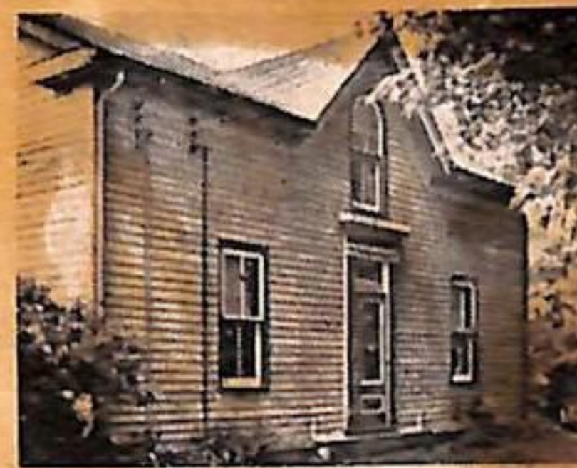
House before restoration.
