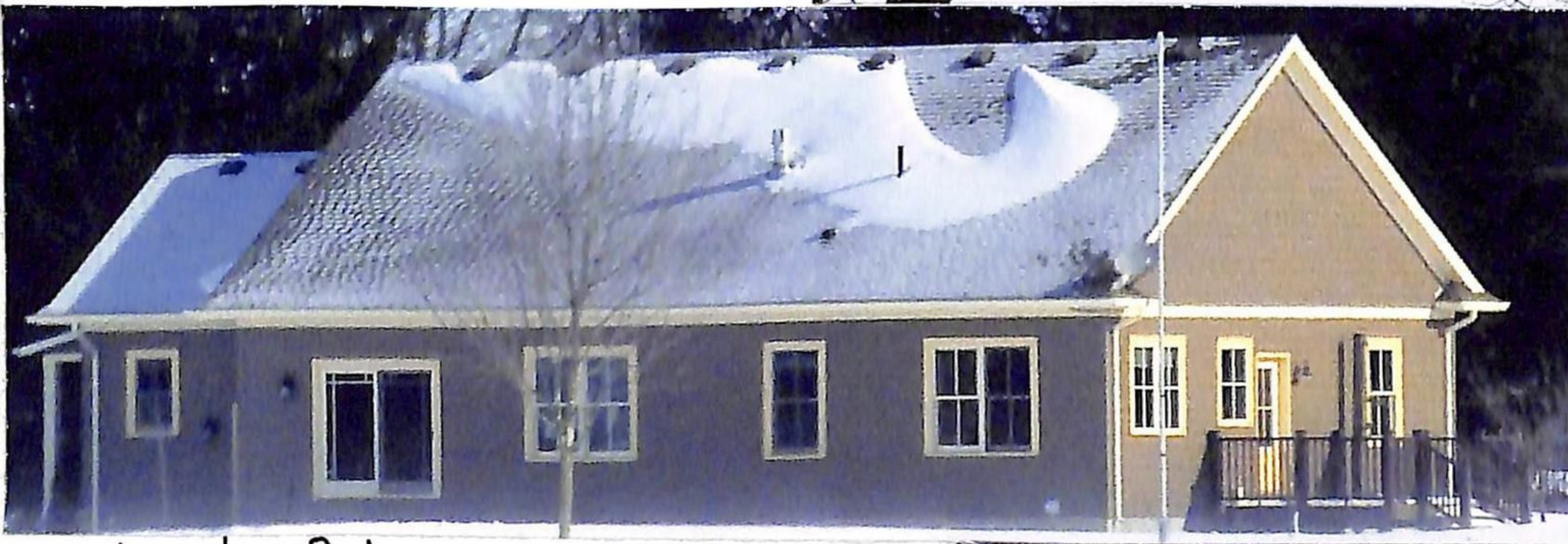
back of house view from Rd. 92
