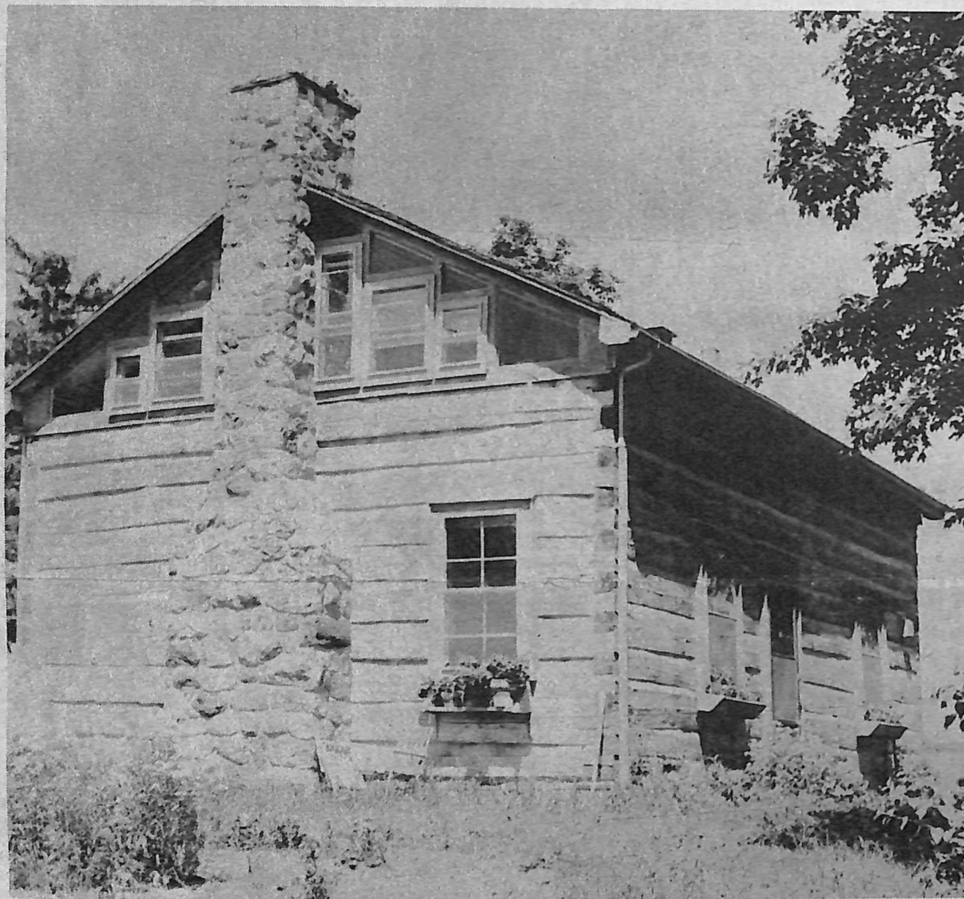
RESTORATION IN WEST MISSOURI — New windows on the upper level, plus a new field stone chimney add much to the charm of this old farmstead along the Thames River, owned by Mr. and Mrs. Bruce Cumming. Note the neat square-hewed dovetail fitting of the rock elm logs at the corners.
