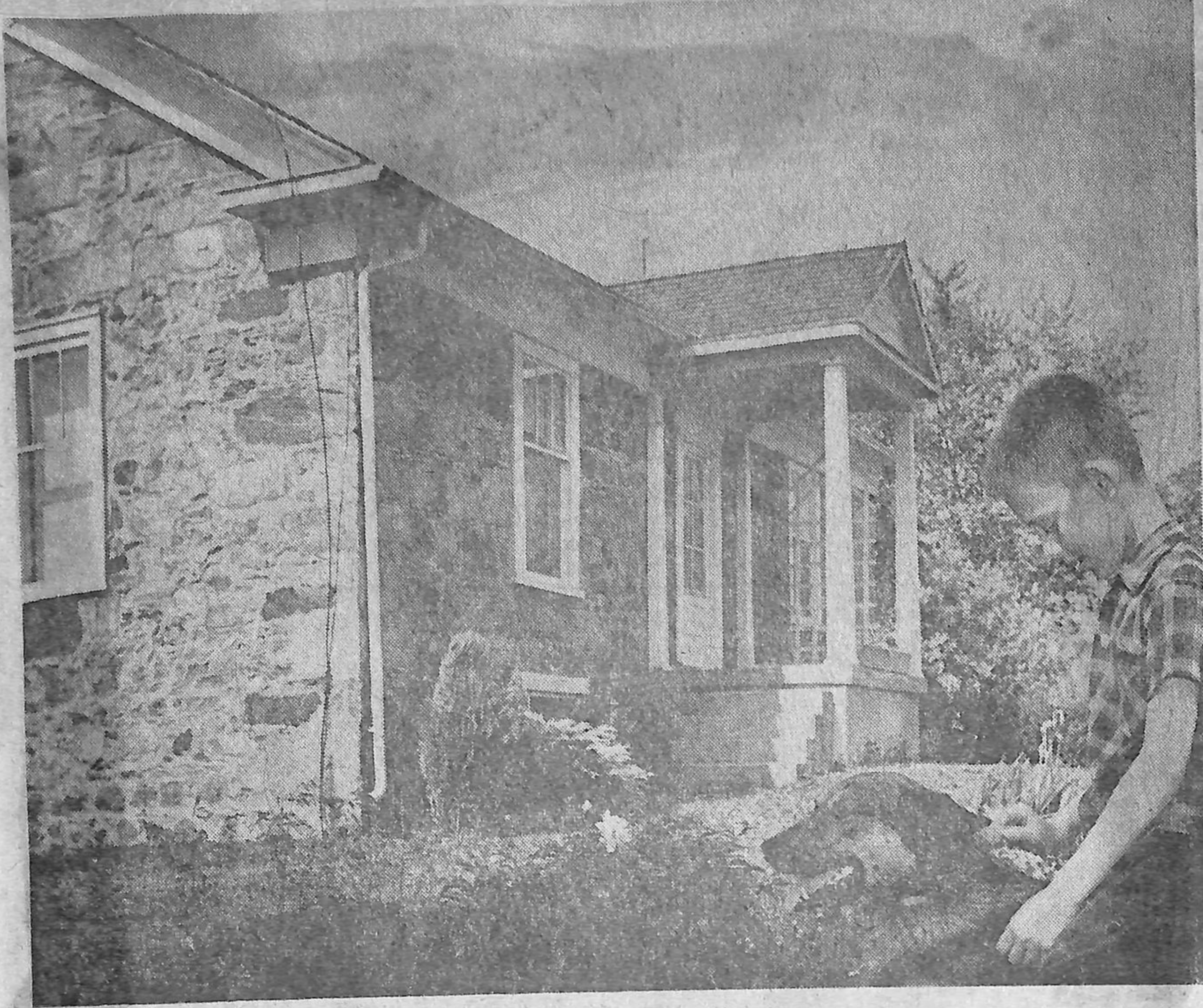
Neil Payne, 7, and Rover are shown beside the Payne home on Highway 2, west of Thamesford. The house, to be torn down in November, has been replaced by a modern ranch-style house.
