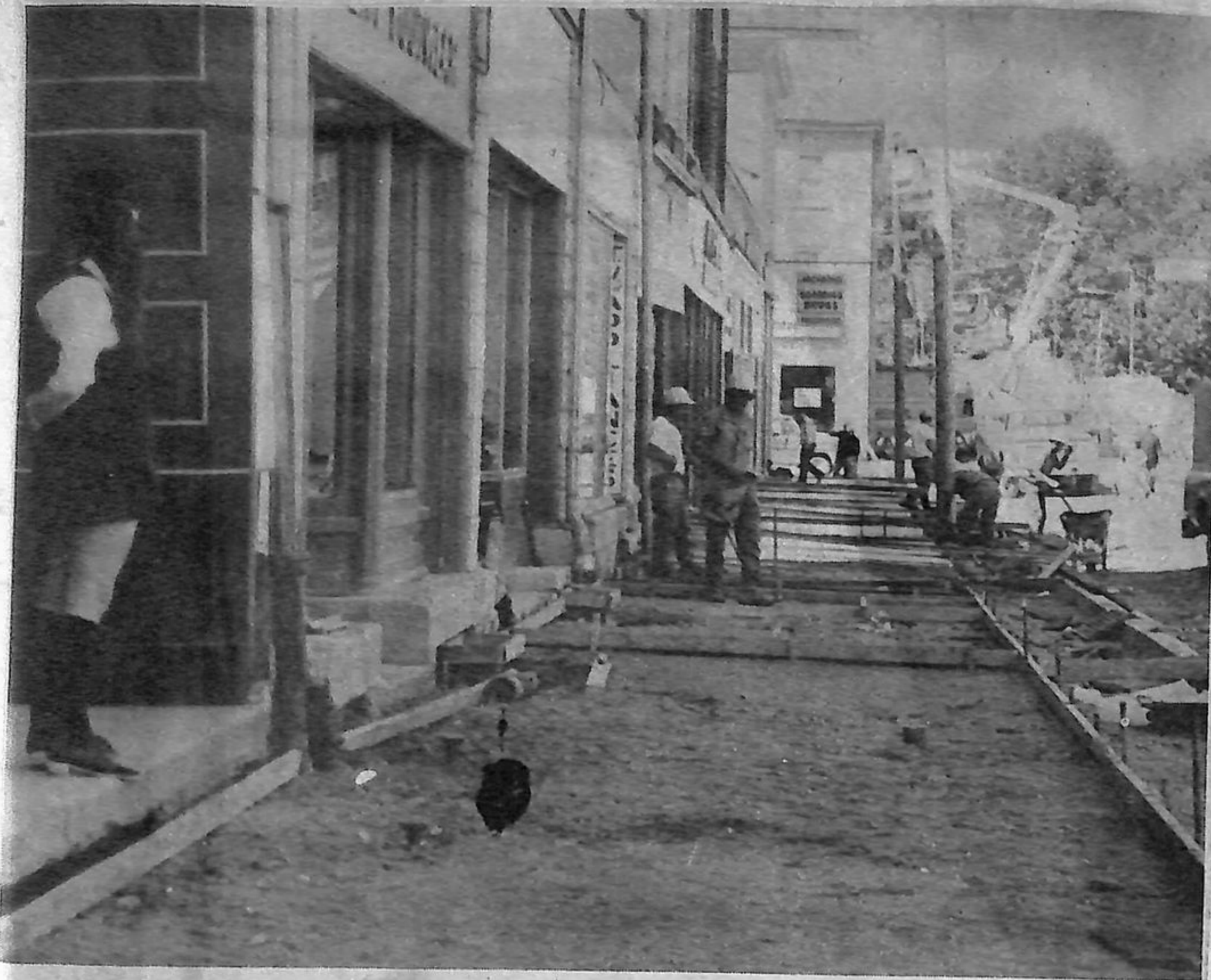
ENCOURAGING STREET SCENE as cement workers install new sidewalks in the downtown area. Small trees, new lamp standards, brick edging and vari-size concrete strips are expected to transform the downtown scene. The wooden poles are temporary installations.
