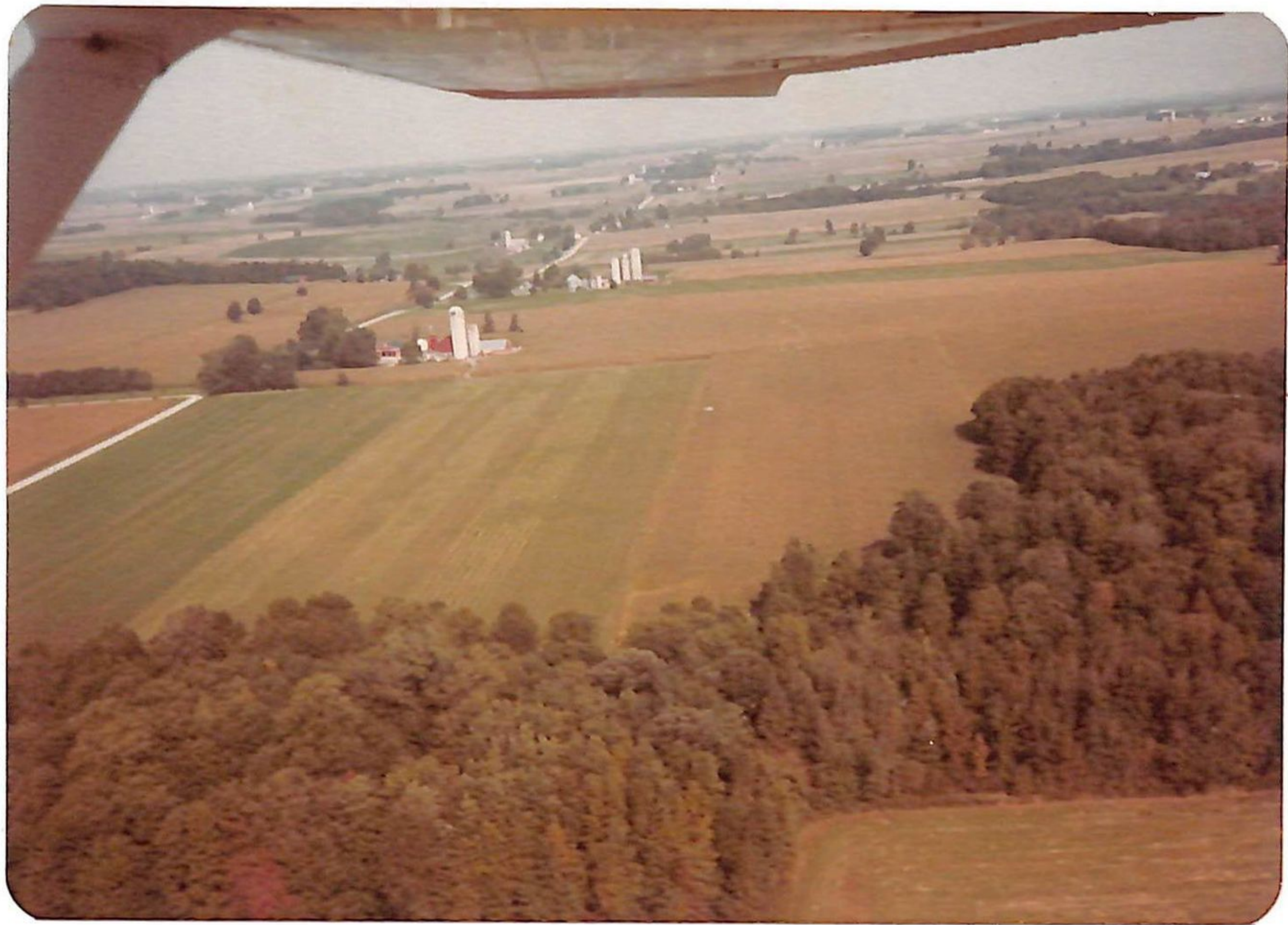
View of Braemar Valley looking north up the 10th Line toward the Braemar Road.
