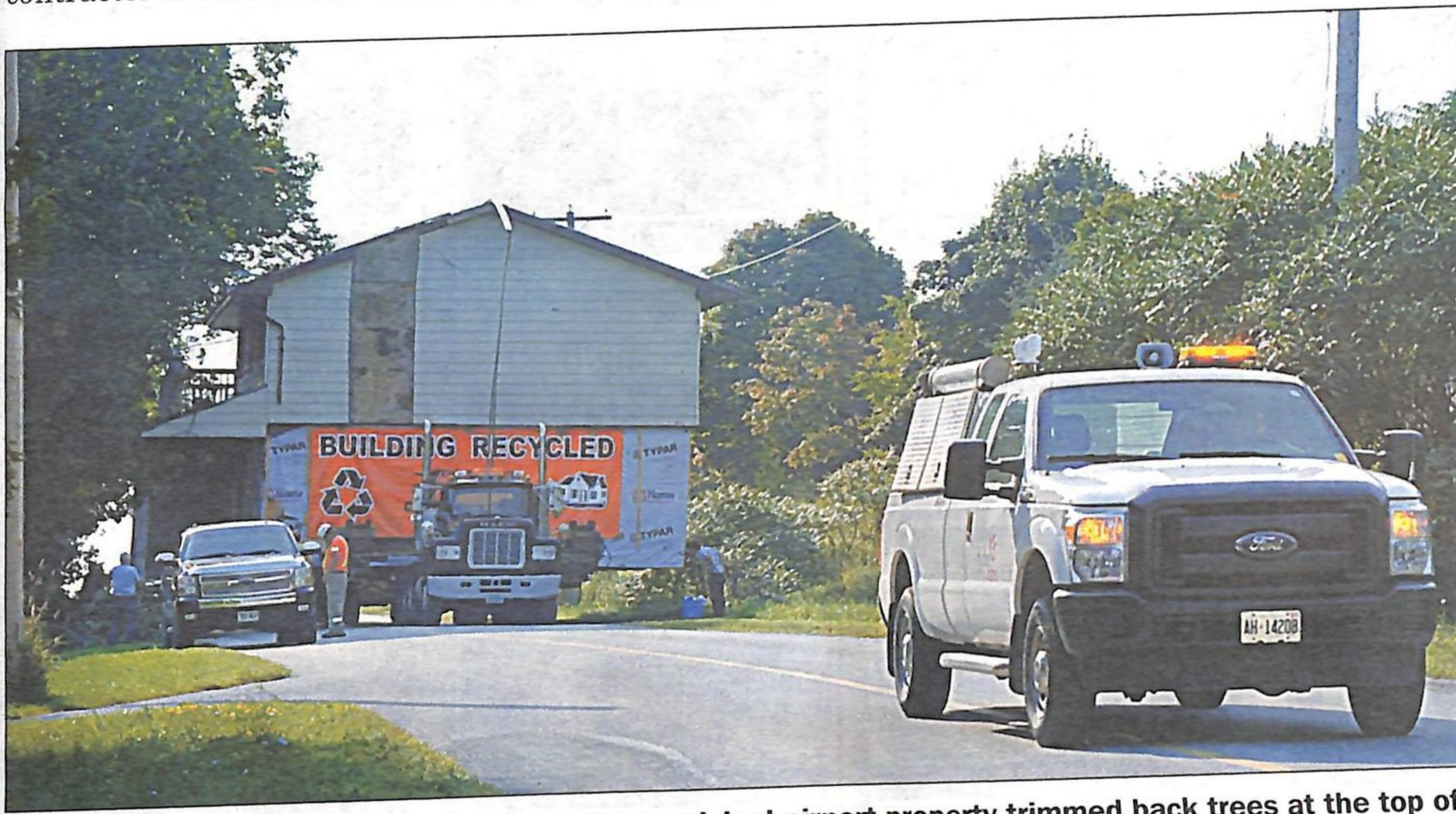
Crews moving the house from the Kincardine municipal airport property trimmed back trees at the top of the hill on Concession 5 to get the wide load through. It will be set on a new foundation on Bruce Road 15. (Barb McKay photo)
