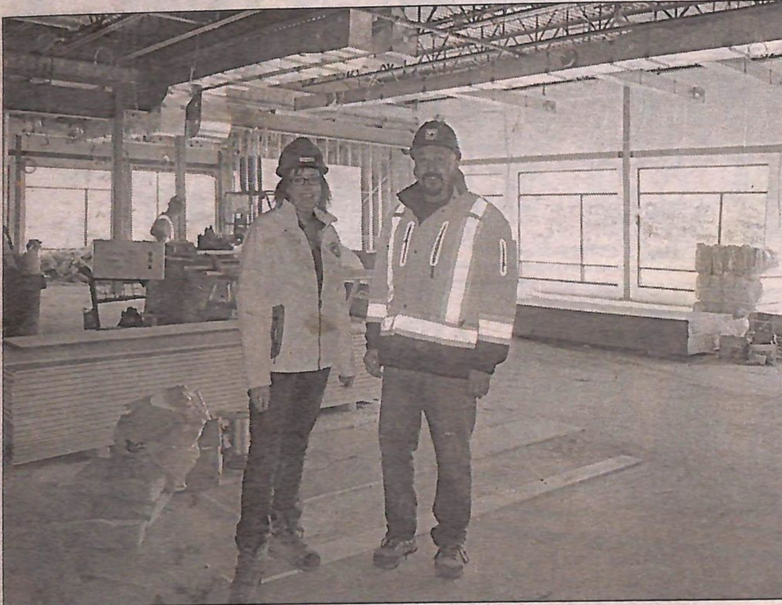
TownePlace Suites general manager Jackie Pawlikowski, left, and site supervisor Bill Rothdeutsch of GUPM stand in what will be the main conference facility in the hotel. (Barb McKay photo)
