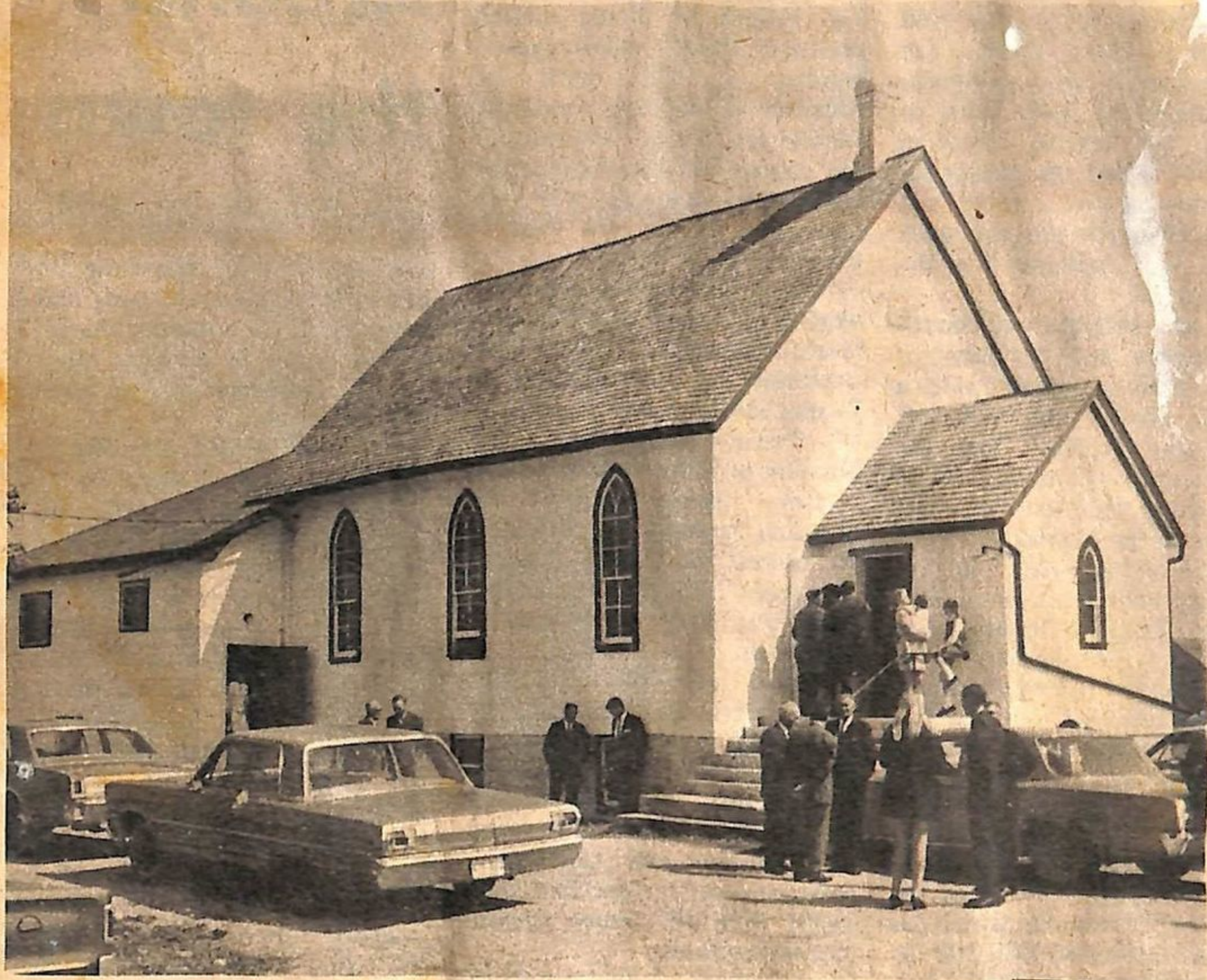
The congregation of the Fourth of Bruce United Brethren Church were proud of the exterior of their building on Sunday as the one hundredth anniversary was celebrated. New siding was recently applied to the church.
