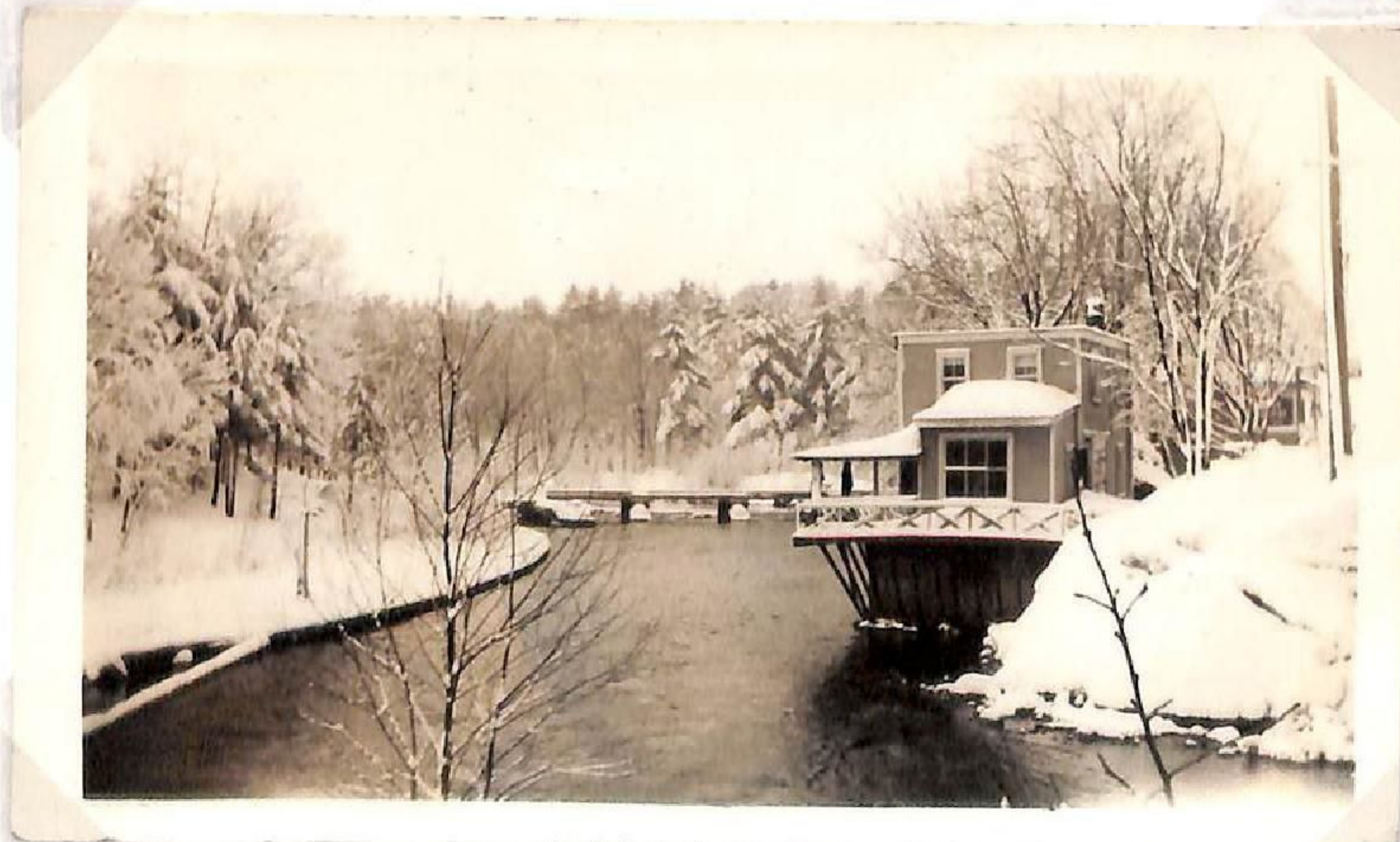
Old telephone office
