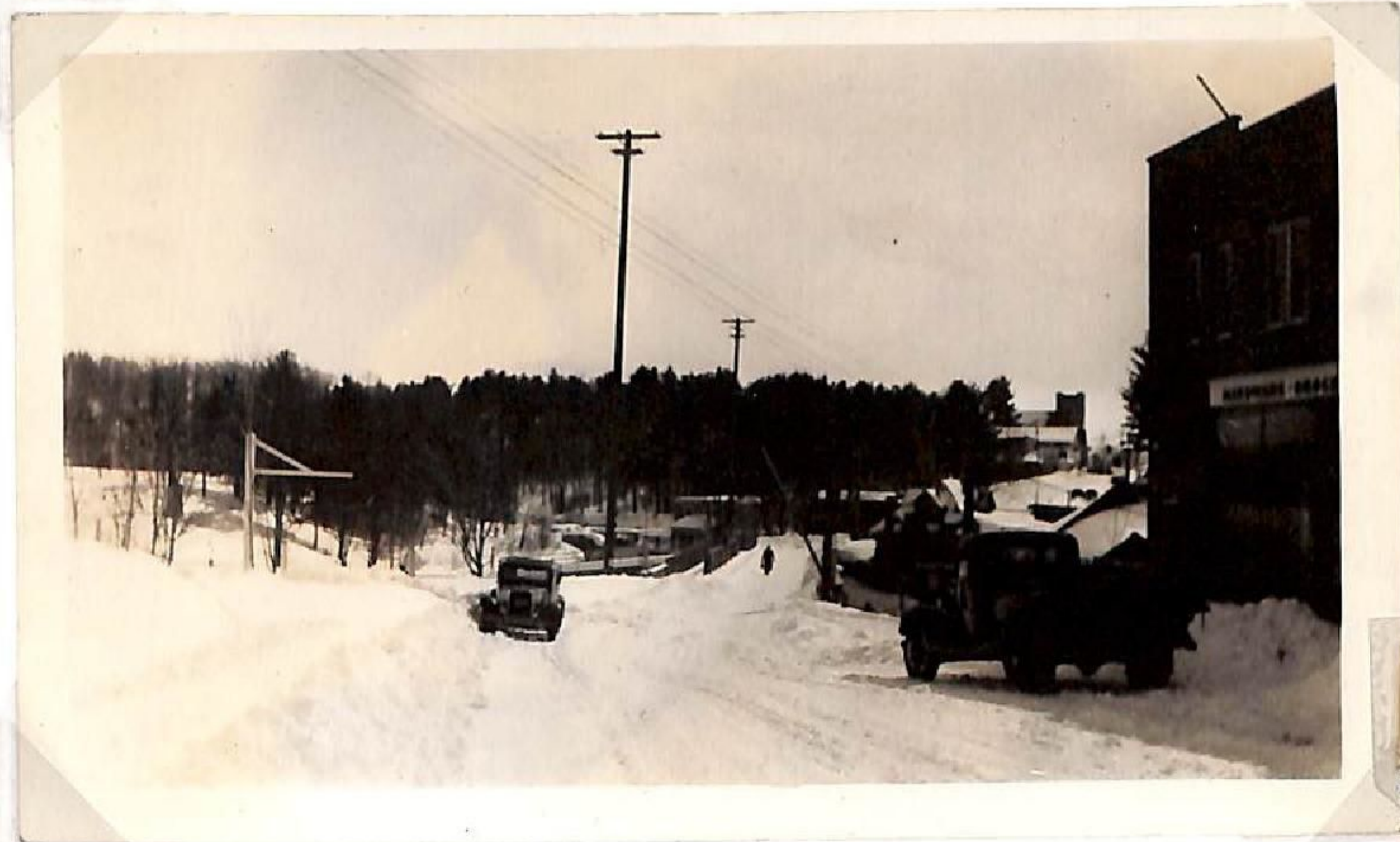
Looking across bridge from Hanna's Store
