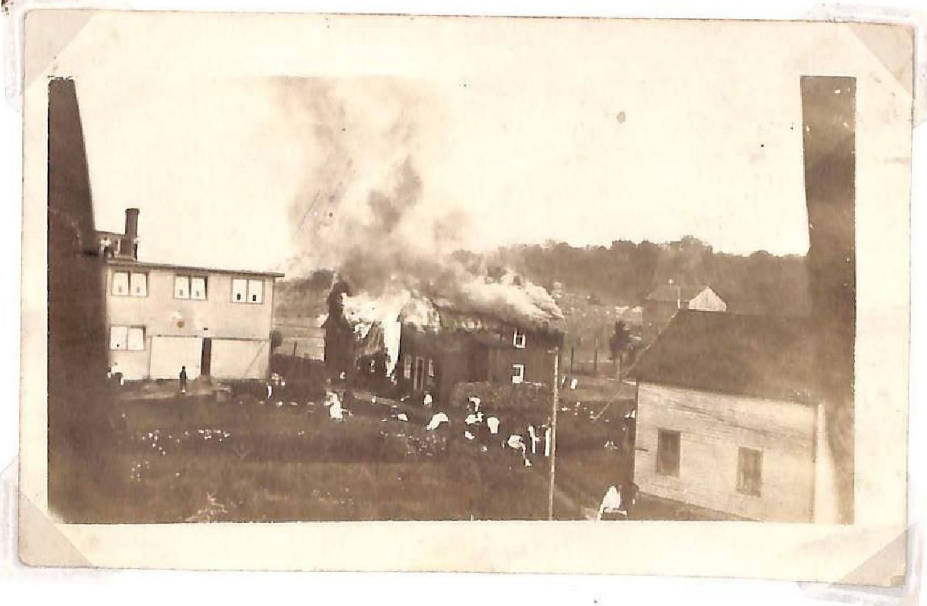
Staffhouse at Elgin House Fire July 1915
