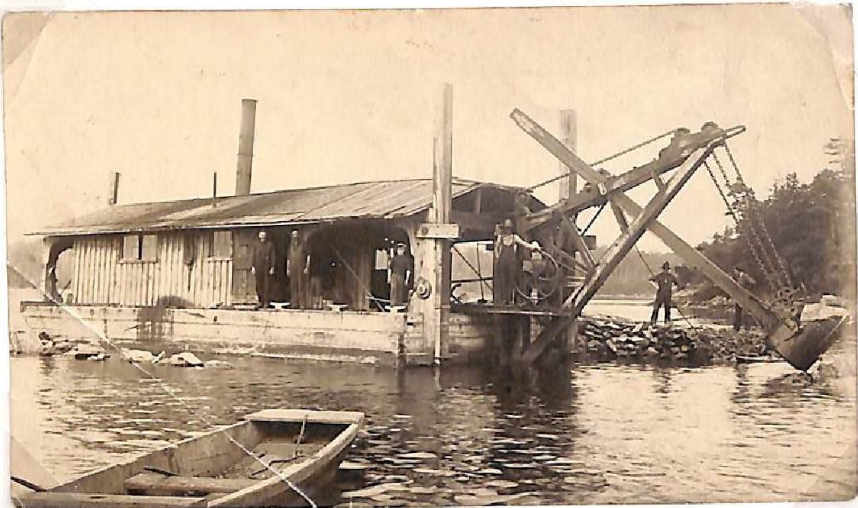
Dredging at small lock (1900+)
