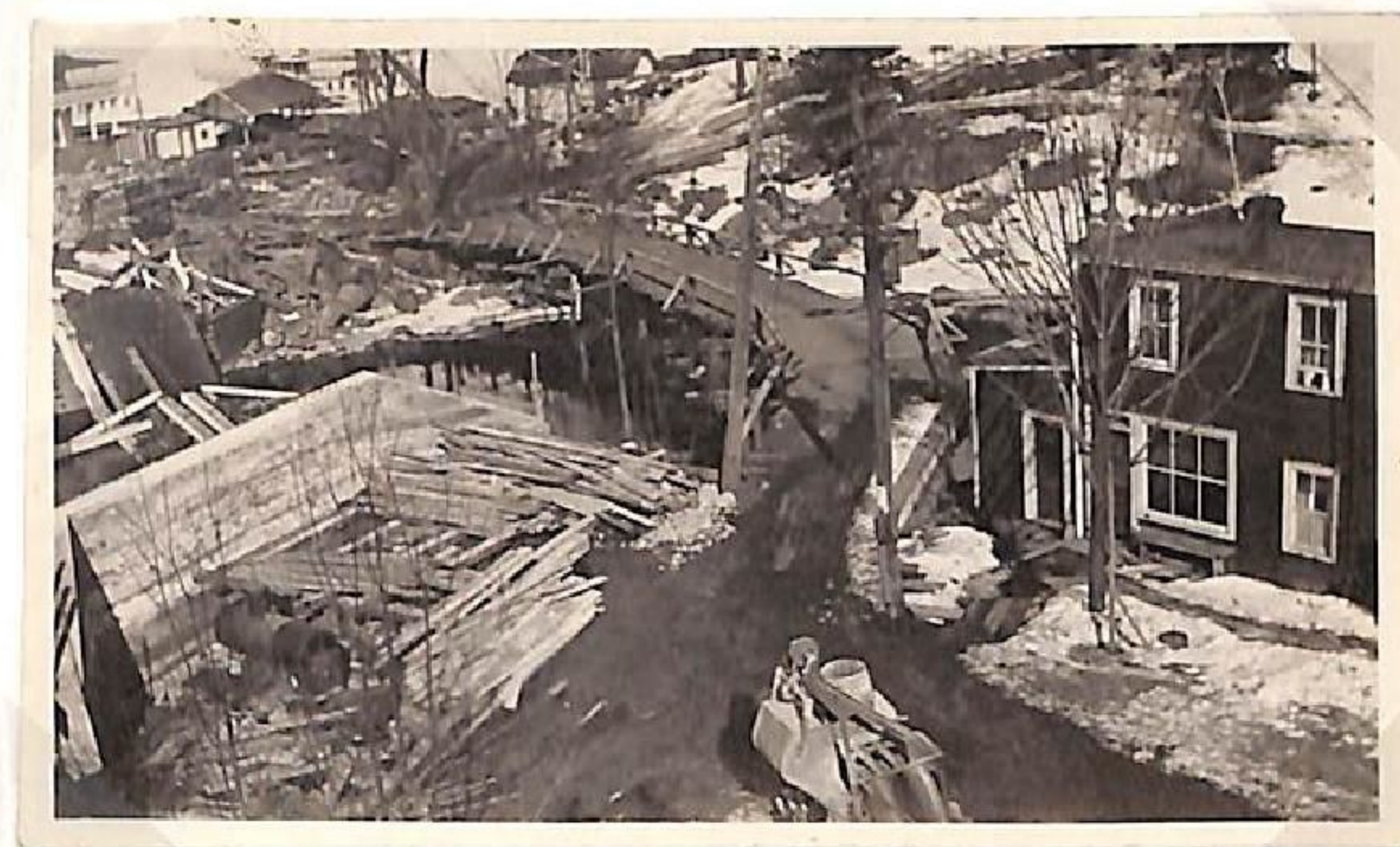
Building New Bridge (1900+)
