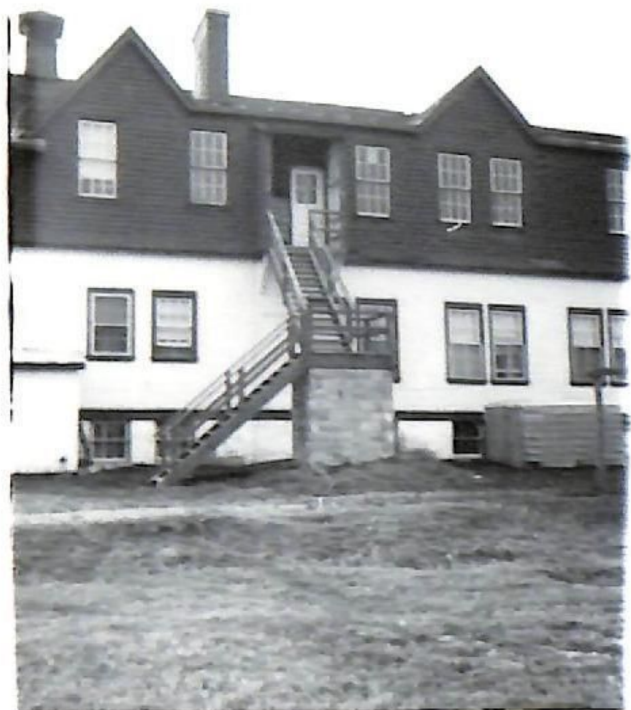
1920-21 Original Dormitory at the Northern Academy, later converted to apts. for Guards families and in 1973, Bldg's demolished to make room for classrooms for A.T.C. class- rooms (in M.C.C.)
