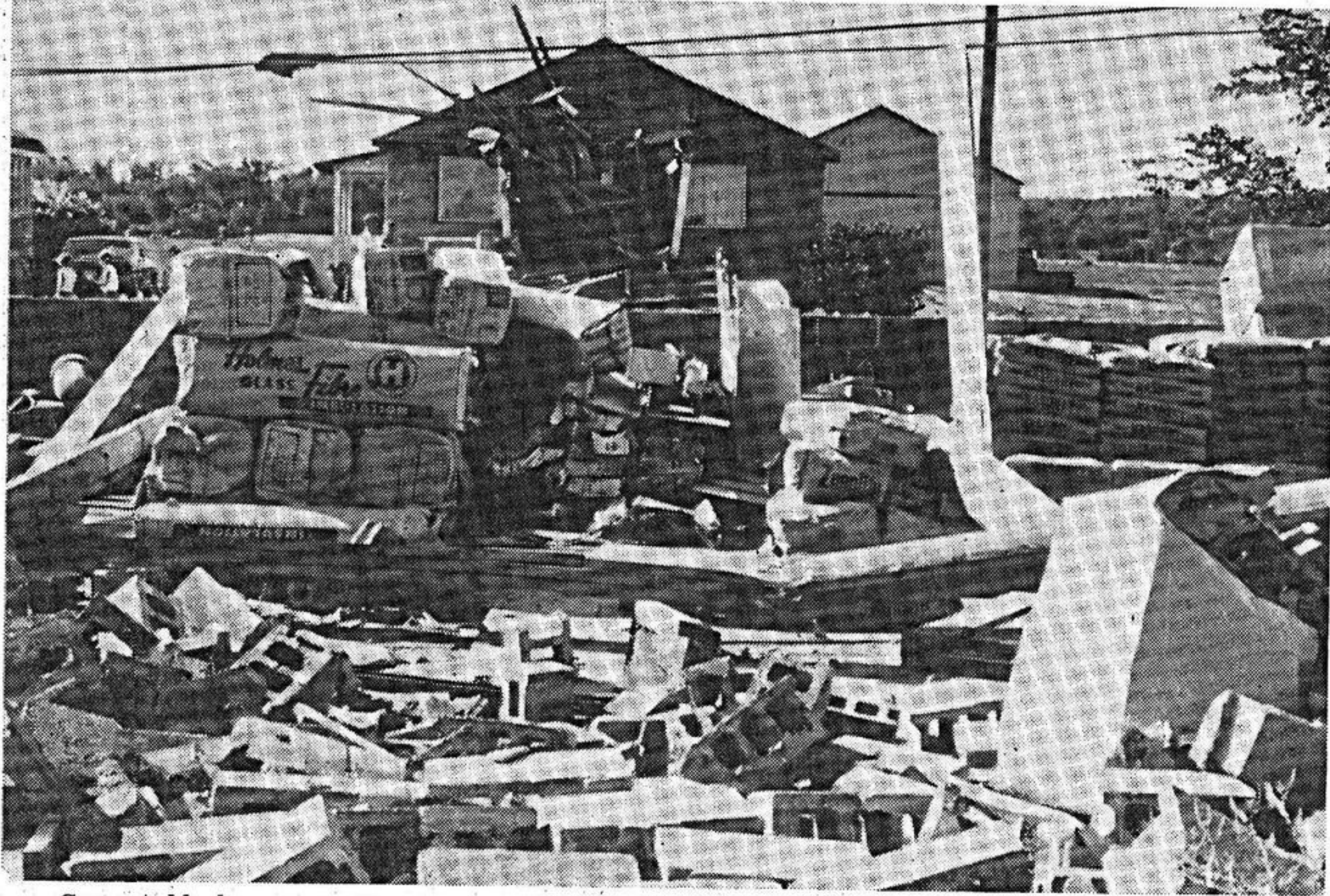
Cement blocks are scattered among building materials at Renfrew Builders Supplies following Saturday evening's freak storm. The damaged house of Leslie White can be seen in the background on the opposite side of the highway.
