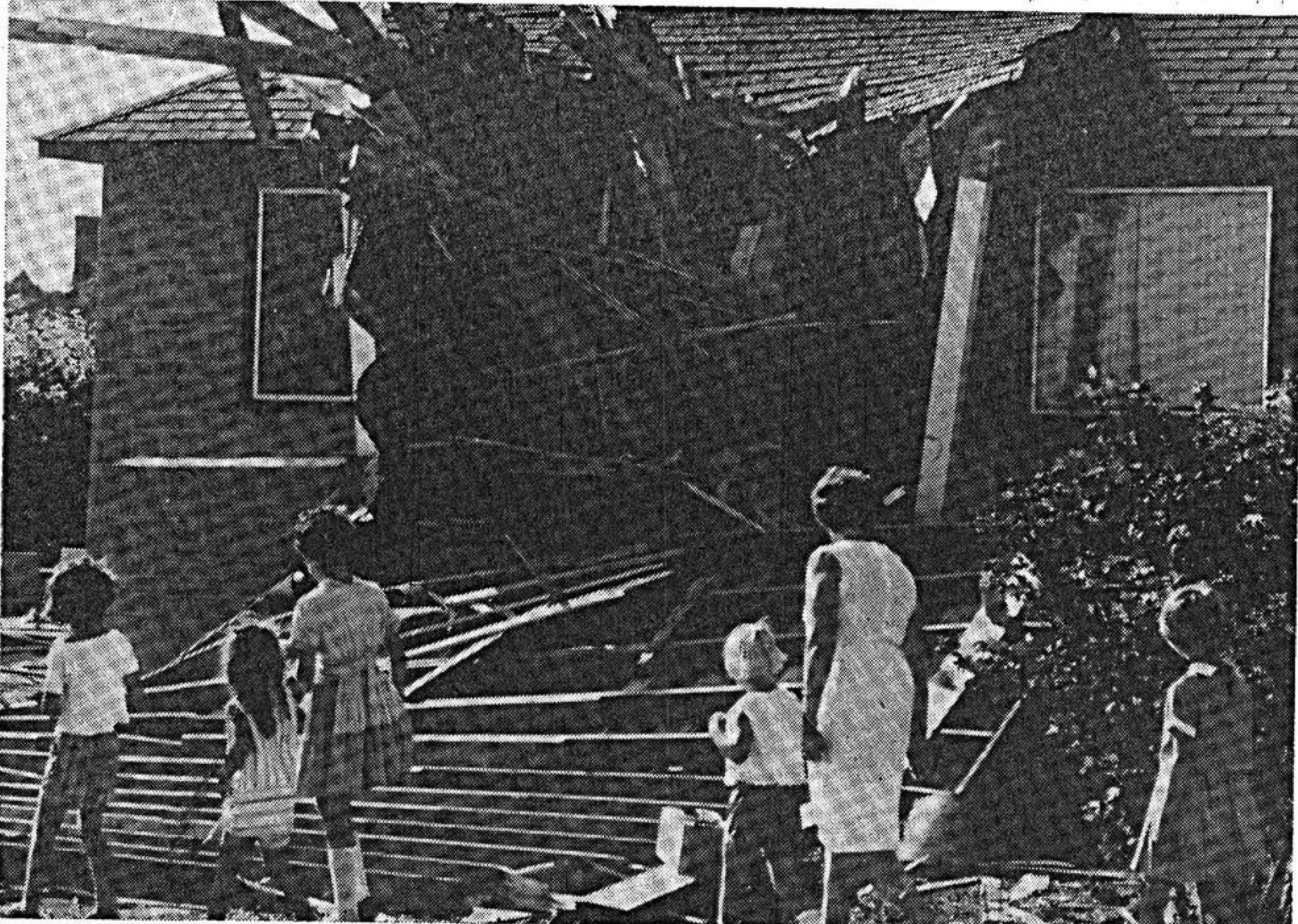
Neighbors view the damaged home of Leslie White. The debris in front of the house is part of the roof of Renfrew Builders Supplies located across the road.
