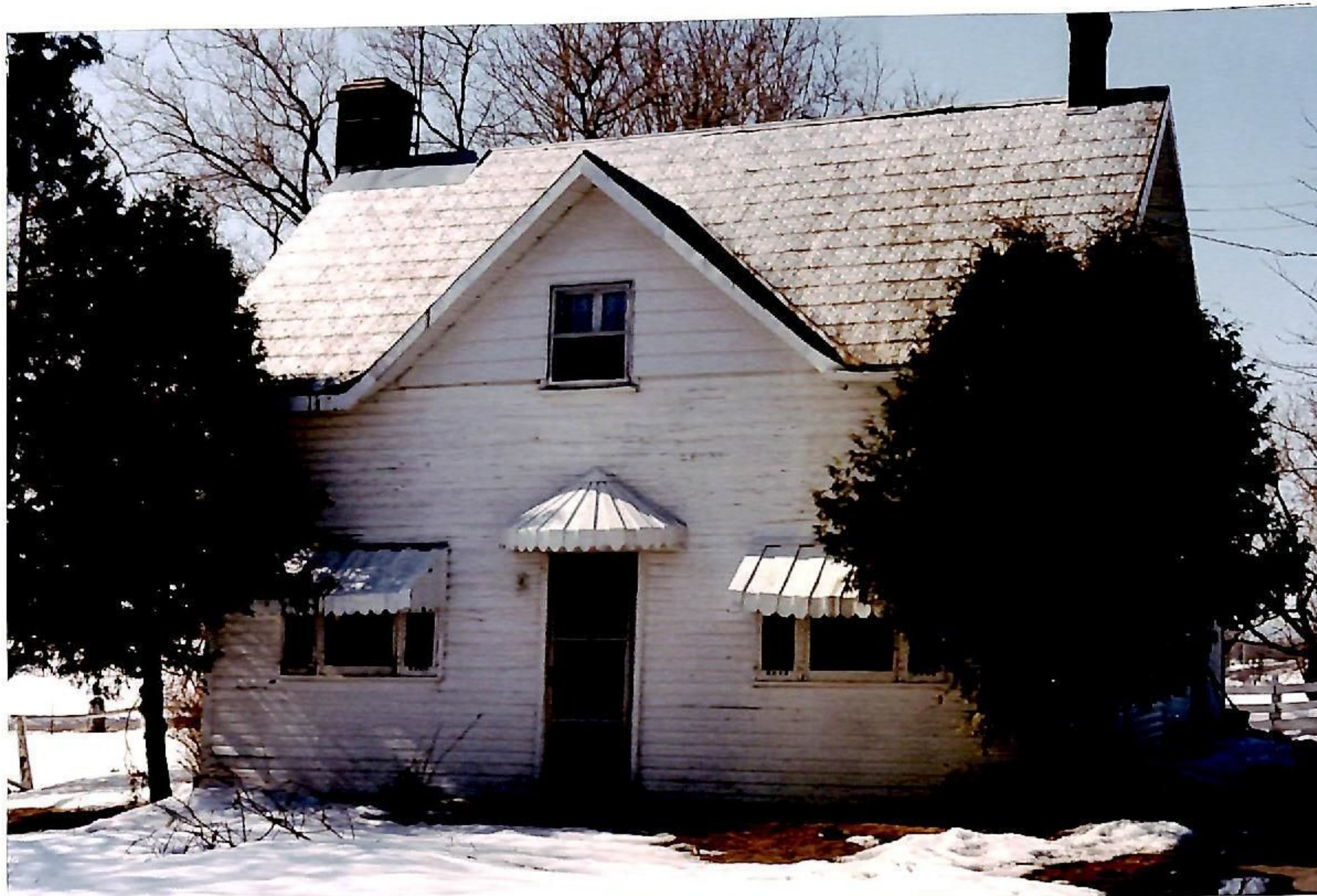
MALWOOD POST OFFICE in 1880's now residence of Allen Kennedy March 1993.
