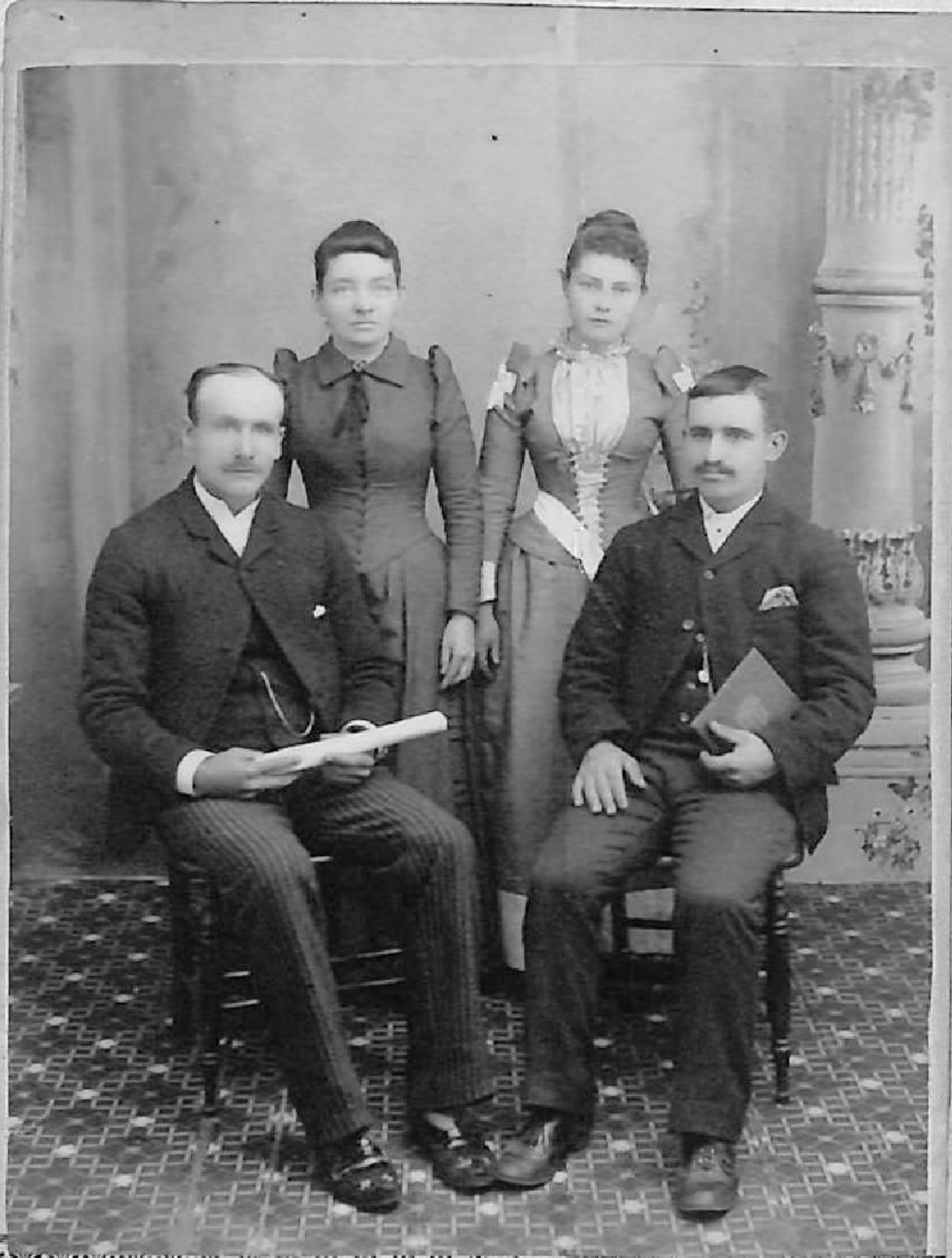
R. W. Ryan, - Photographer, BRACEBRIDGE, ONTARIO.
