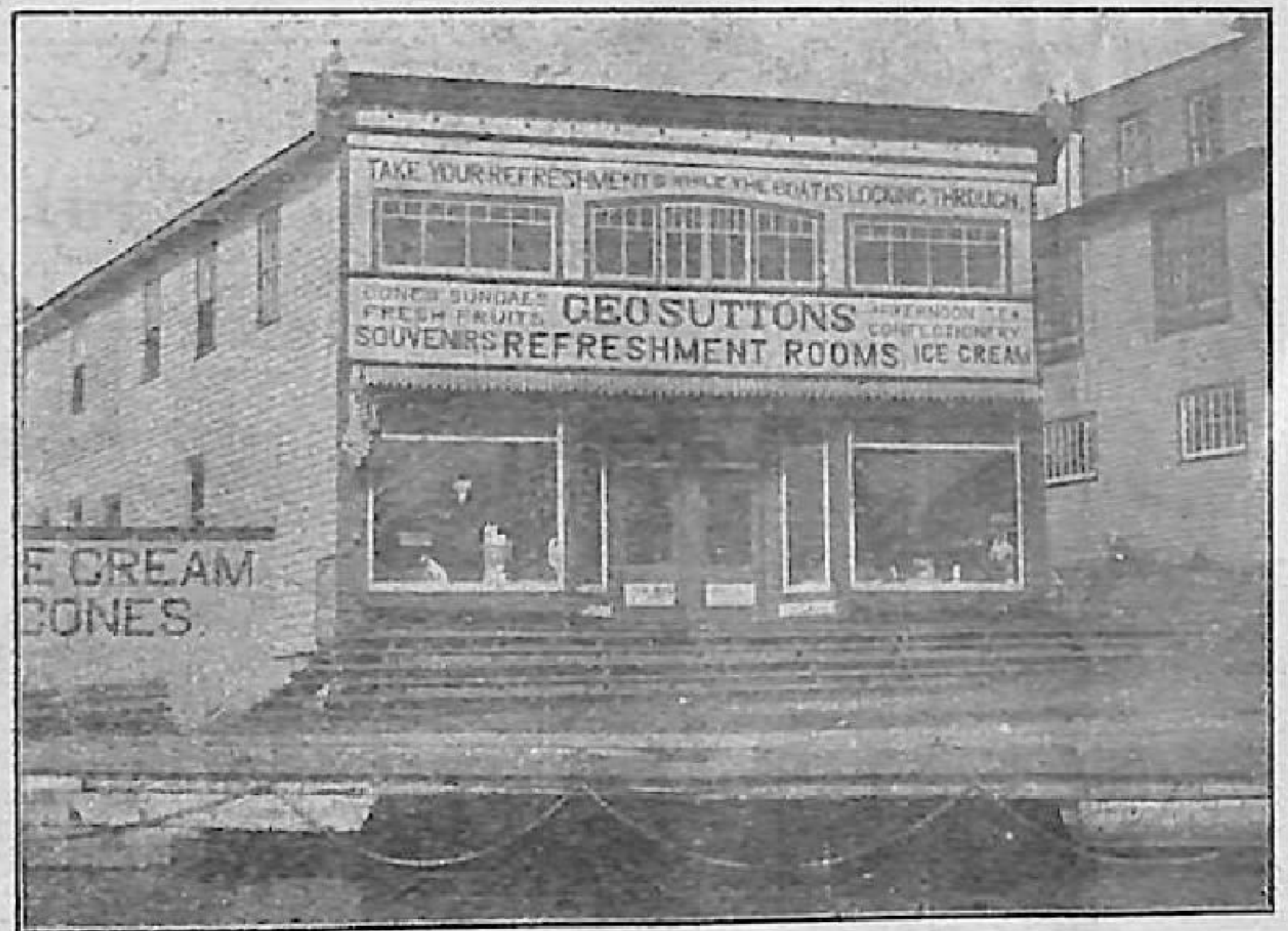
In the great fire of October, 1931, Sutton's Ice Cream Parlor and Dance Hall was burned to the ground along with many other buildings. The 21 Club occupies the site now where the building stood — one of the first buildings to be seen in the business section as the traveller by Lakes steamer arrived at Port Carling coming from Lake Muskoka. The building was erected about 1914. Mr. George Sutton had previously operated an ice cream business as well as a butcher shop, located near the locks from 1888 until 1907, and then on the main street, until the above building was erected.
