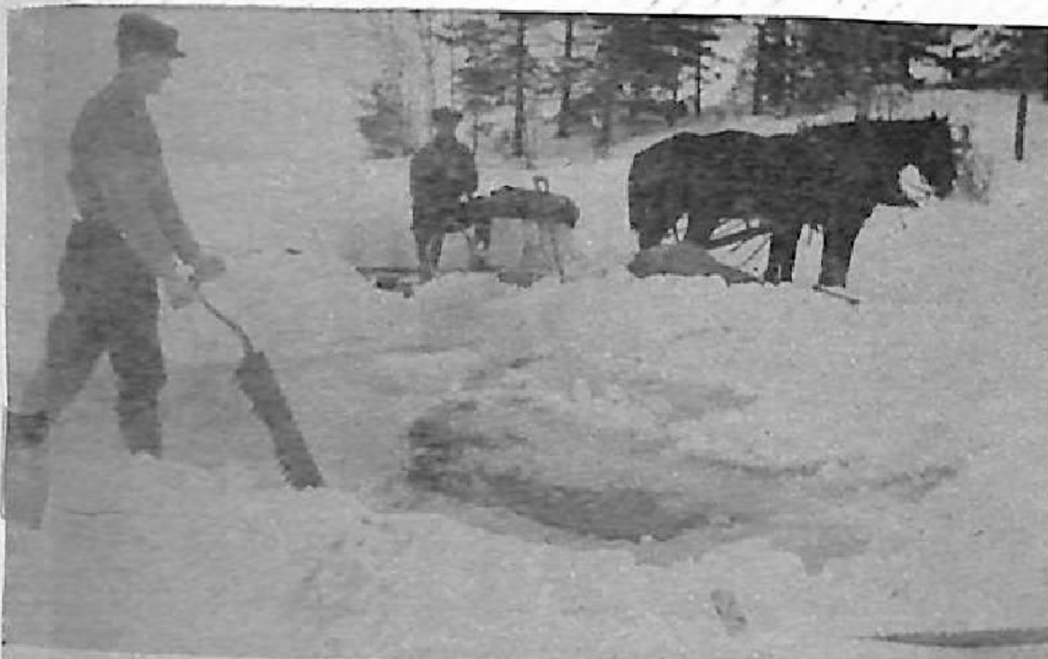
CUTTING ICE: Before electric refrigeration, many summer locations had ice houses from which ice could be sold to cottagers for their "ice box" refrigerators. The ice was cut from the lake during the winter in large blocks and stored, covered with sawdust, in well built and well shaded buildings.
