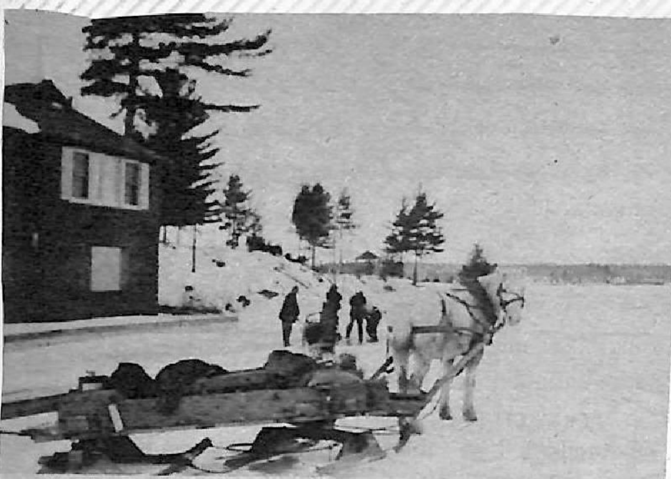
ICE FOR SAFETY'S SAKE: The men are busy cutting through the ice in front of the wharf to protect it from the ice movement in the spring breakup. The location was where the late Colonel Moodie had his summer home at the Lake Rosseau outlet into the Indian River.
