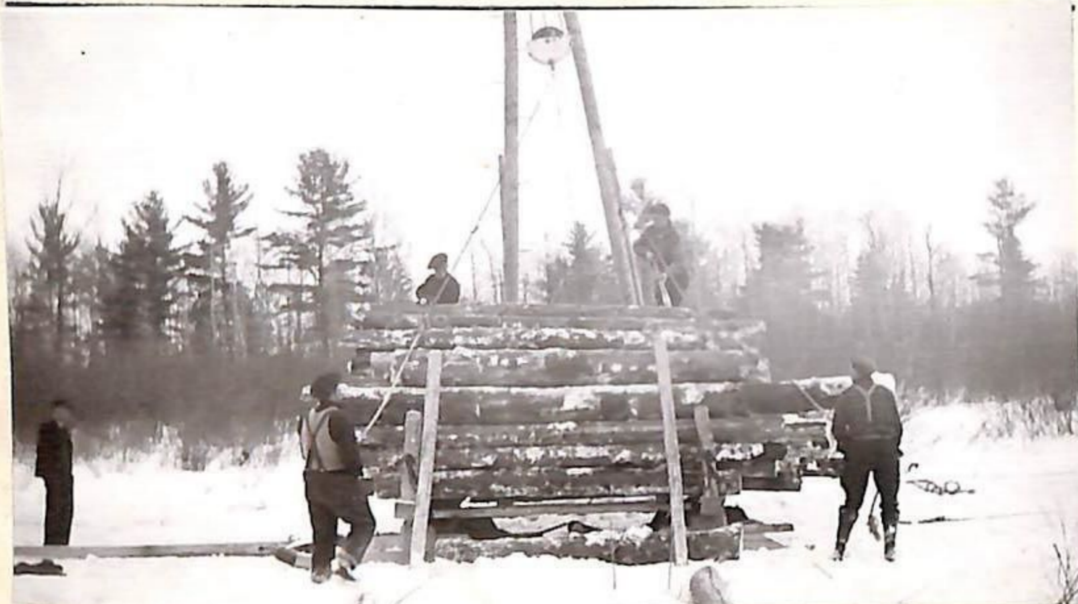
P.W.SHAW - Logging operations at West Arm Limit
