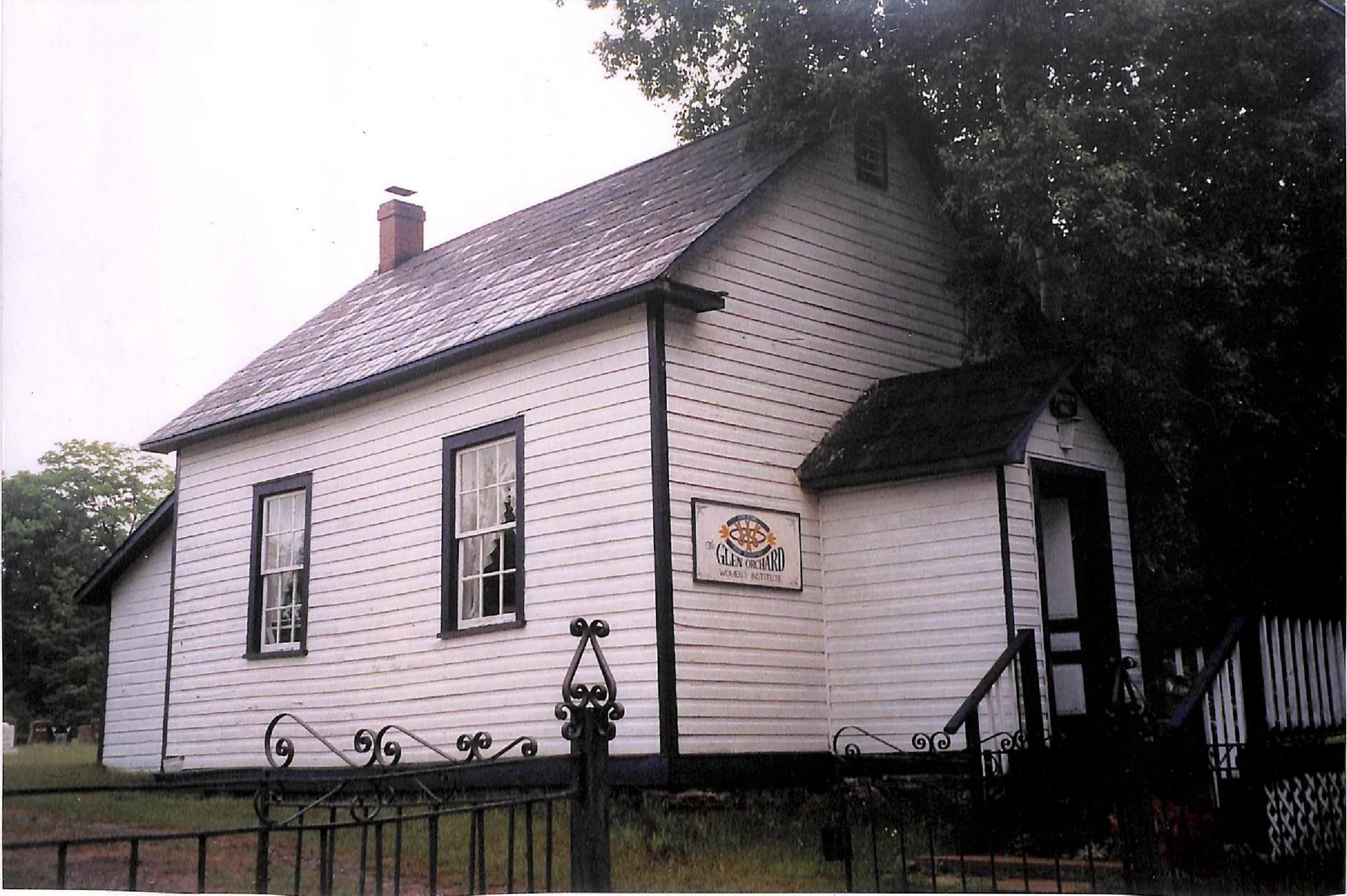
OLD SCHOOL HOUSE 1890 BEFORE BEING RESTORED.
