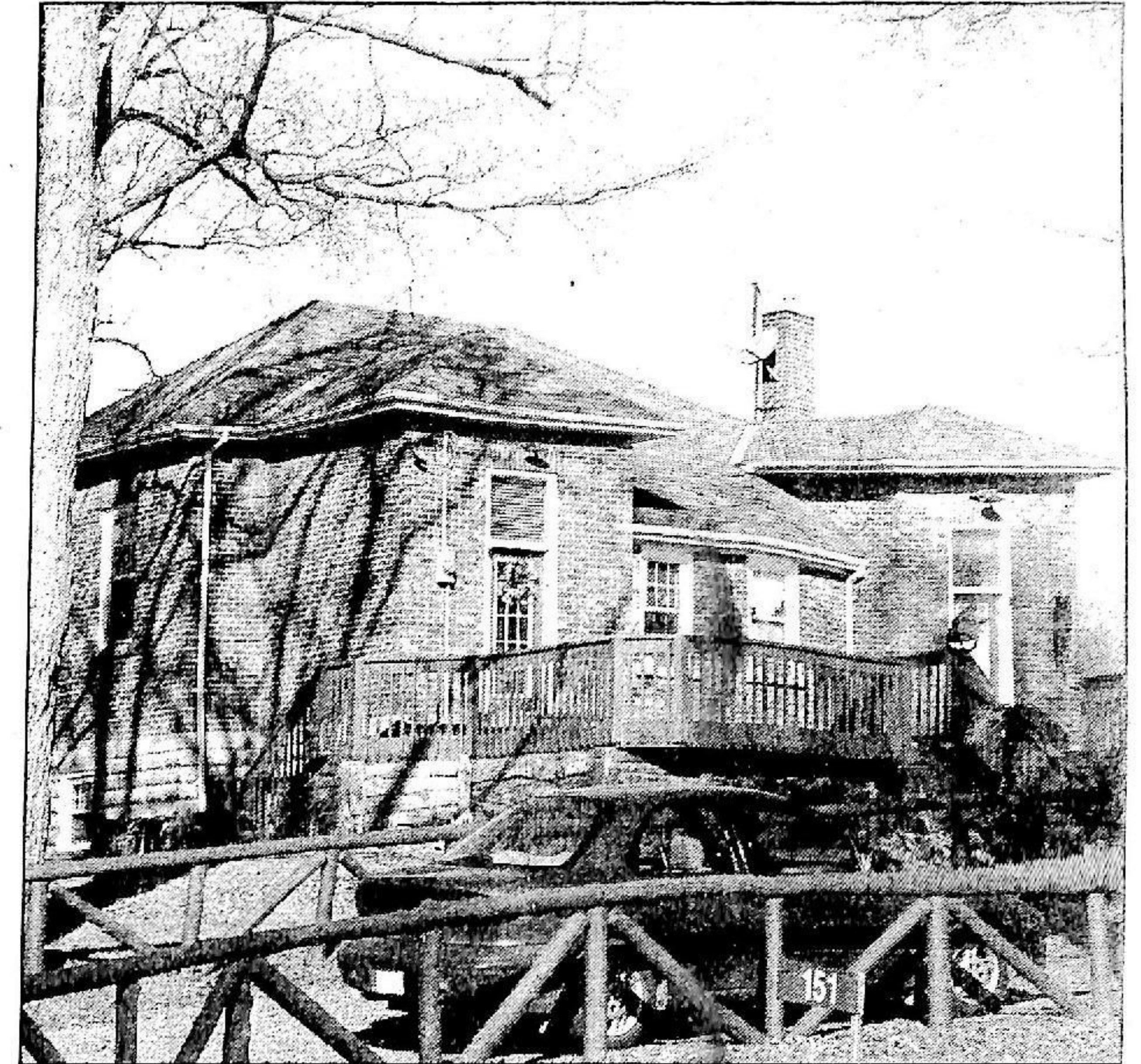
This Castleton school was noteworthy for its white-painted tin ceiling and basement furnace (as opposed to the usual box stove in the middle of the classroom area).
