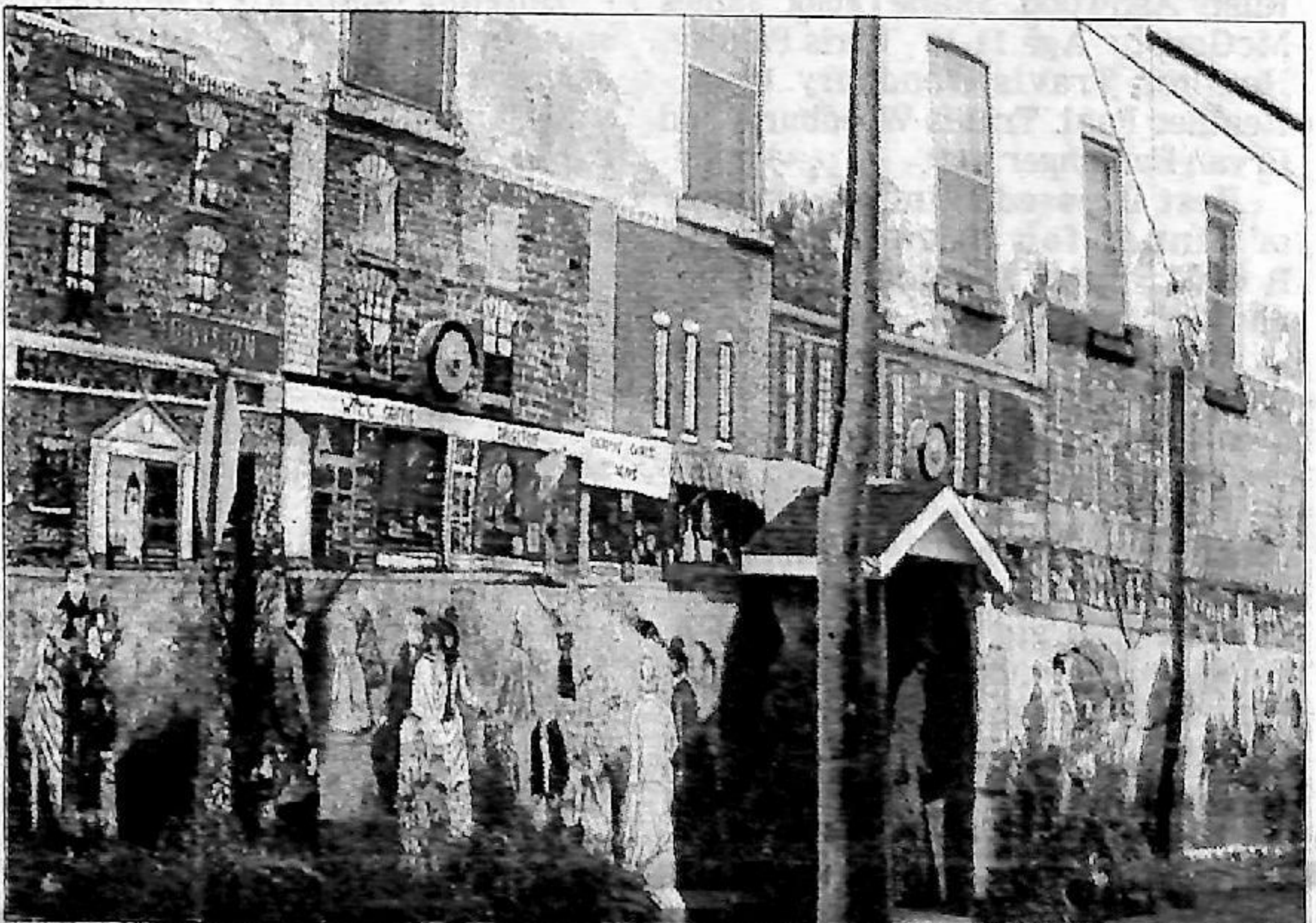
The mural on the east wall of the Queen’s Hotel in Colborne fronts on Division Street South.
