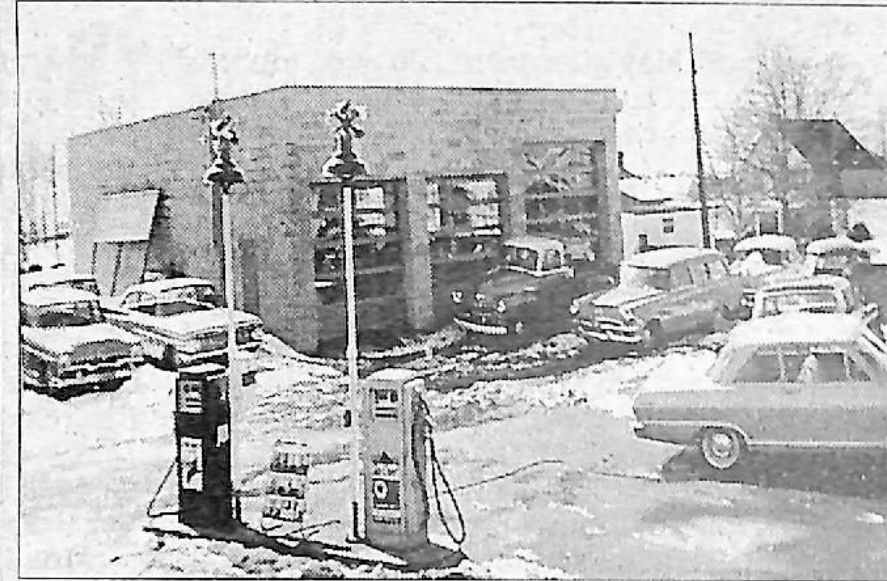
1961: Three new cement block service bays were built by local builder Charlie Teal at 17 Toronto Road - one large enough to accommodate trucks.
