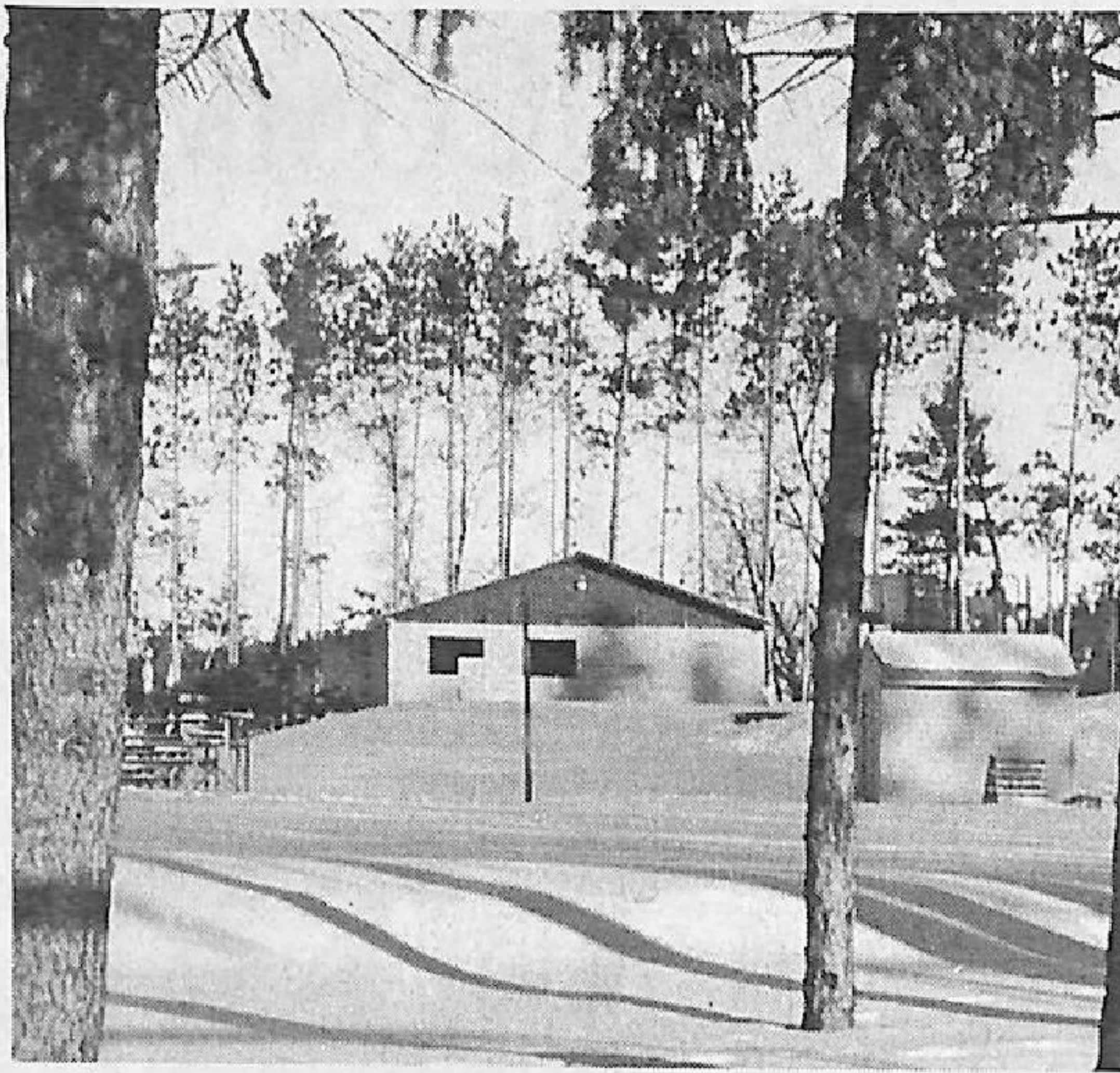
The new canteen and washroom facilities are slated for spring opening
