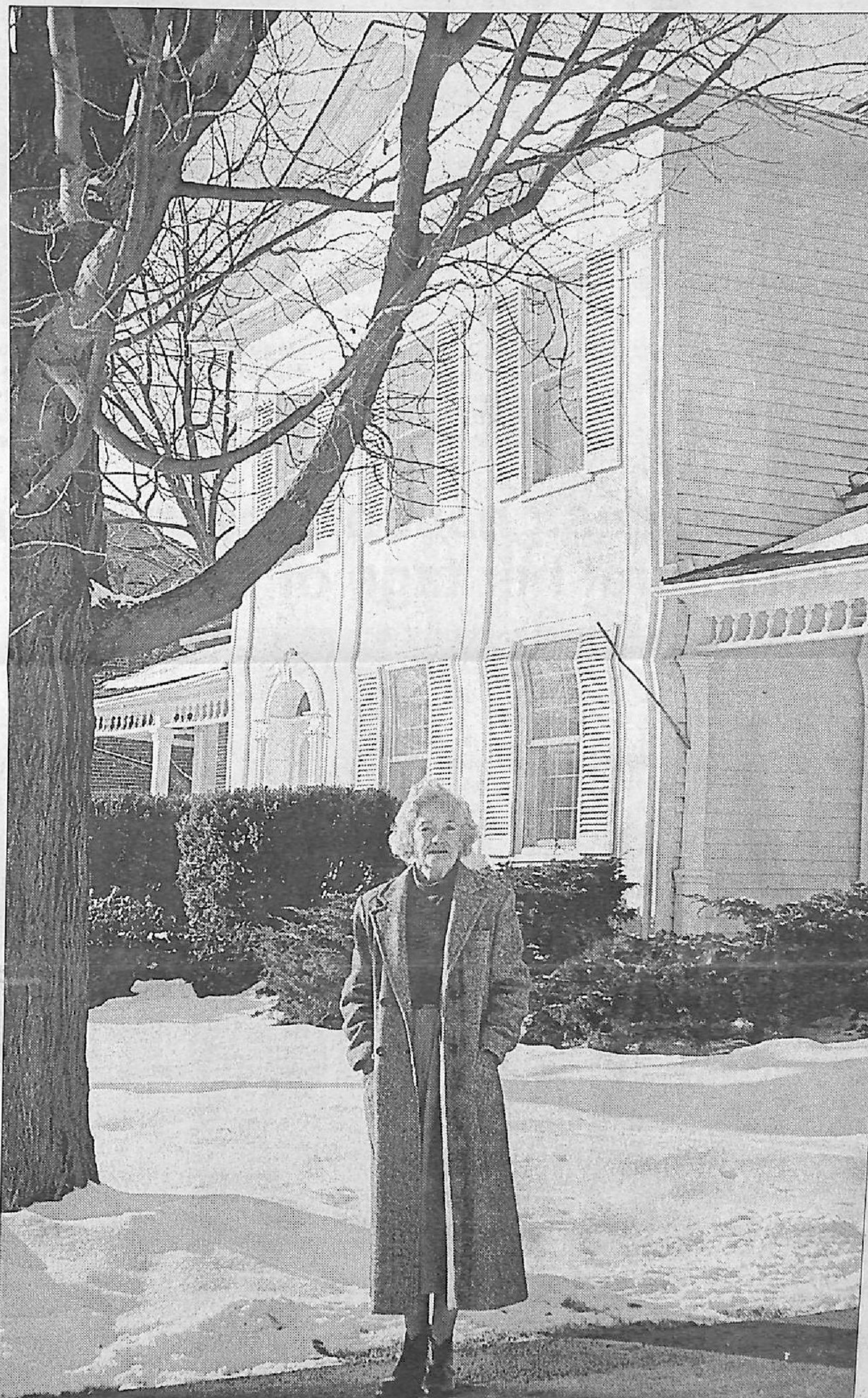
The jewel in the crown of Colborne architecture is the Keeler homestead at 9 Church Street West. Marian Carter has asked the home be designated to ensure the historical and architectural heritage of the home she and her husband, the late Nick Carter, treasured is preserved for future generations. See story on page 2.
