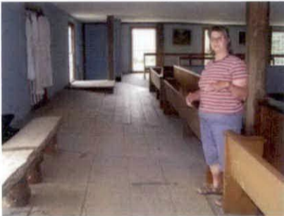
Darlene Johnston, in upper level of Hay Bay Church, points out the gallery effect with use of a downward floor slope.
