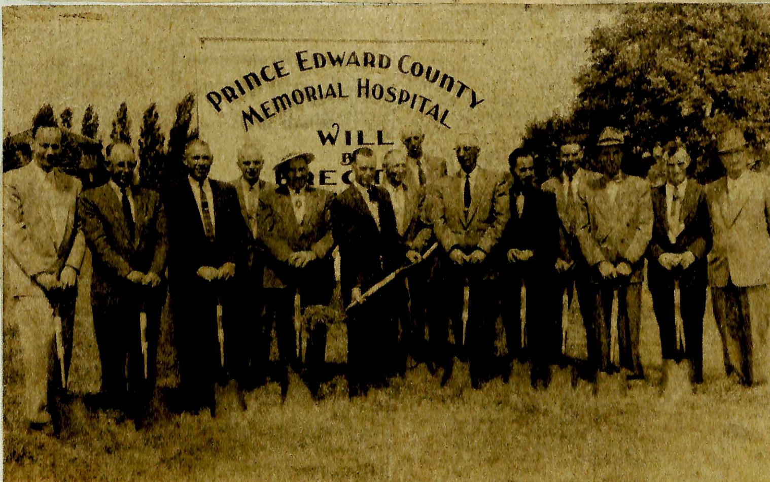
A joyous moment came Wednesday morning for officials of Prince Edward County Hospital Board when members of County Council turned the sod for the new $600,000 memorial hospital. It is expected construction on the new modern building will be started this fall. County Councillors shown in the above Hodgson
