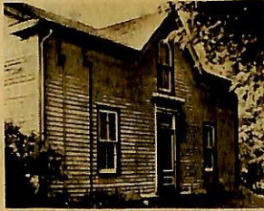
House before restoration.
